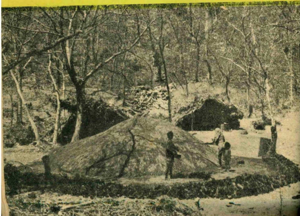
Wood unsuitable for use as timber is turned into charcoal. A kiln being worked at Maswan (Thana District), also on co-operative lines.
