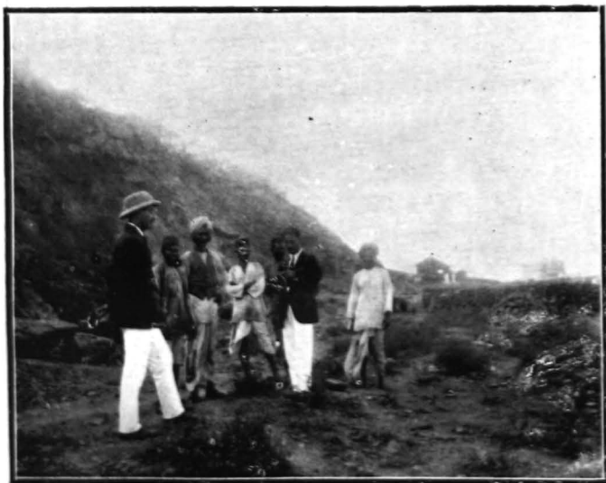
Mr. Nariman on inspection of B. D. D. works in suburbs.
