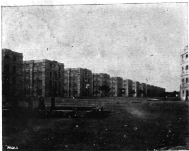
A long line of unoccupied Chawls at Worli.
