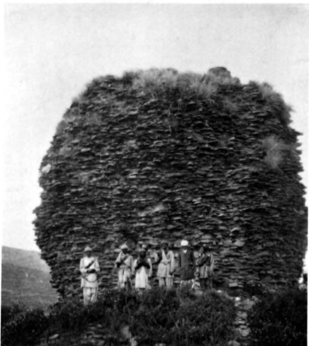
42. RUINED STŪPA STRIPPED OF ITS MASONRY FACING, NEAR CHĀRRĀGH.
