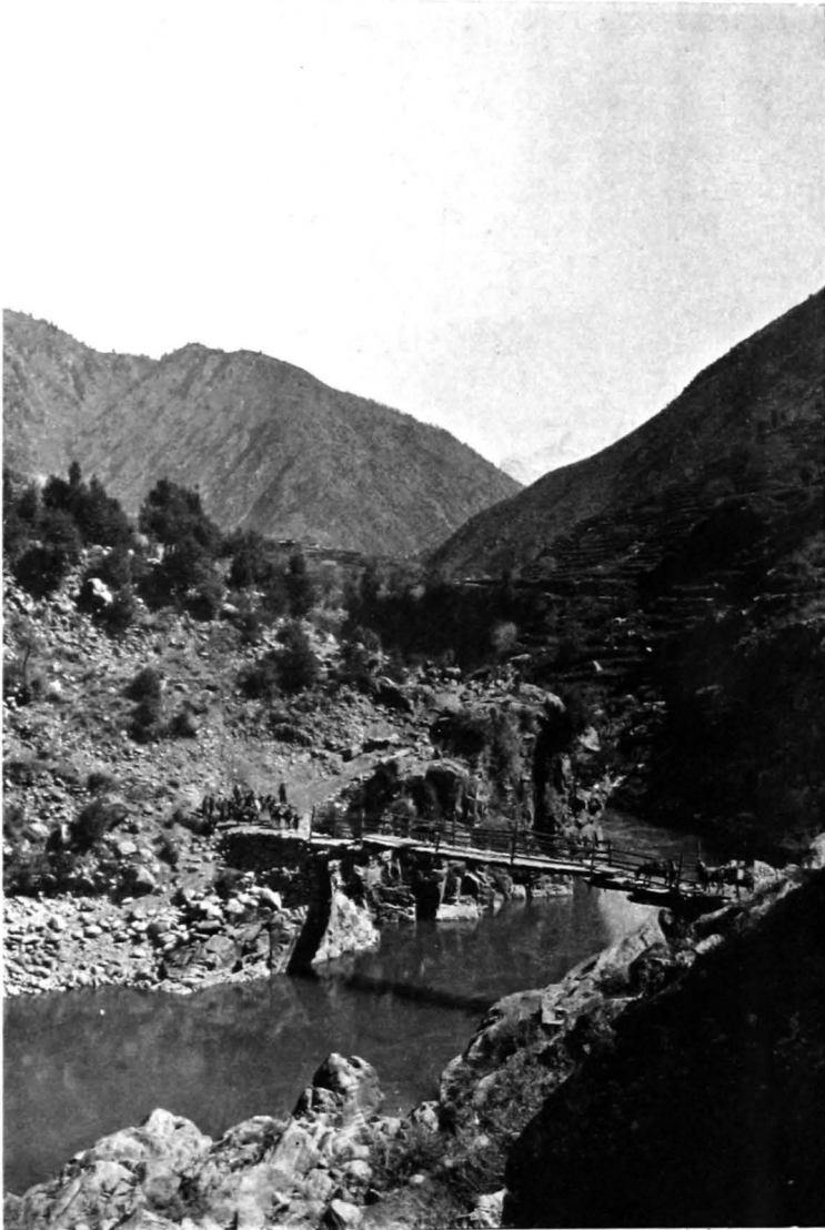
51. BRIDGE OVER SWĀT RIVER AT AĪN, BELOW BRANIĀL.
