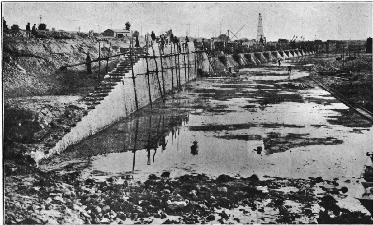
SUKKUR BARRAGE WORKS.
