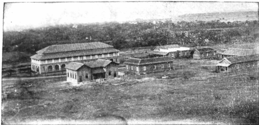
The Servants of India Society's Buildings. (View from the adjoining hill.)
