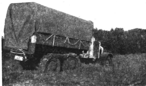
A SINGLE CHAIN TRACK VEHICLE IN USE IN SOFT MUD.
