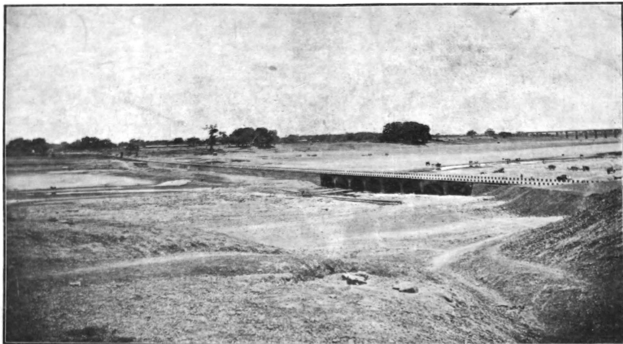
Sholapur District. Causeway over the river Bhima at Pandharpur.
