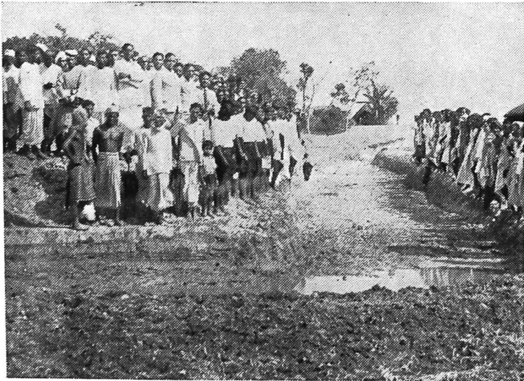
THE ABOVE SCENE SHOWS THE OPENING OF A khal OR WATER-CHANNEL, EXCAVATED BY VOLUNTARY LABOUR. HUNDREDS OF SUCH khals HAVE BEEN EXCAVATED IN BENGAL DURING THE PAST TWO YEARS AS PART OF THE MINISTRY'S RURAL RECONSTRUCTION DRIVE, LOCAL OFFICIALS INSPIRING ENTHUSIASM FOR THE WORK ON A VOLUNTARY BASIS AMONG THE LOCAL POPULATION.
