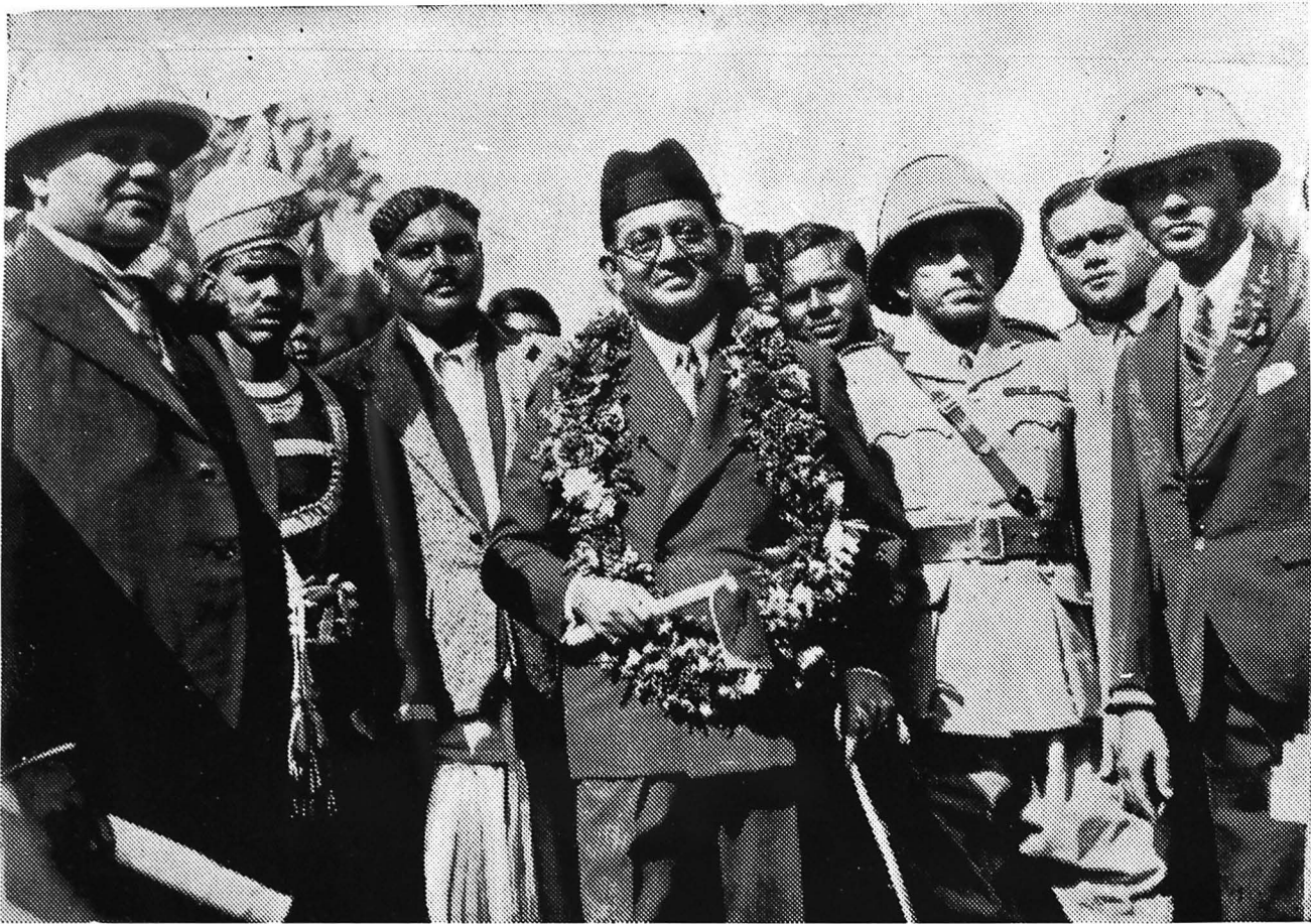
THE HON'BLE MAHARAJA S. C. NANDY, MINISTER FOR COMMUNICATIONS AND WORKS, ABOUT TO TURN THE FIRST SOD OF THE BHAIKAB CUT, AT JESSORE.
