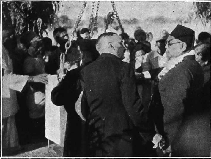
HON'BLE MR. A. K. FAZLUL HUQ LAYING THE FOUNDATION STONE OF THE DACCA AGRICULTURAL INSTITUTE.
