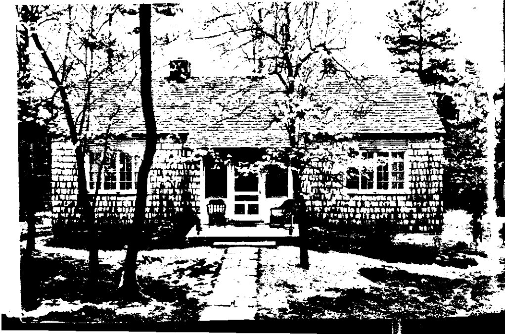
An Example of a Norris House of Frame Construction
