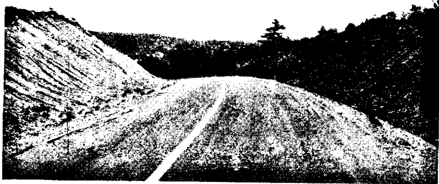
Courtesy The Roadside Bulletin Ugly, Steep, Raw Banks Left Untouched after Road Construction
