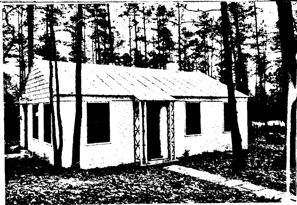
A Small, Cinder-block House. One of TVA's Significant Contributions to Low-cost Housing
