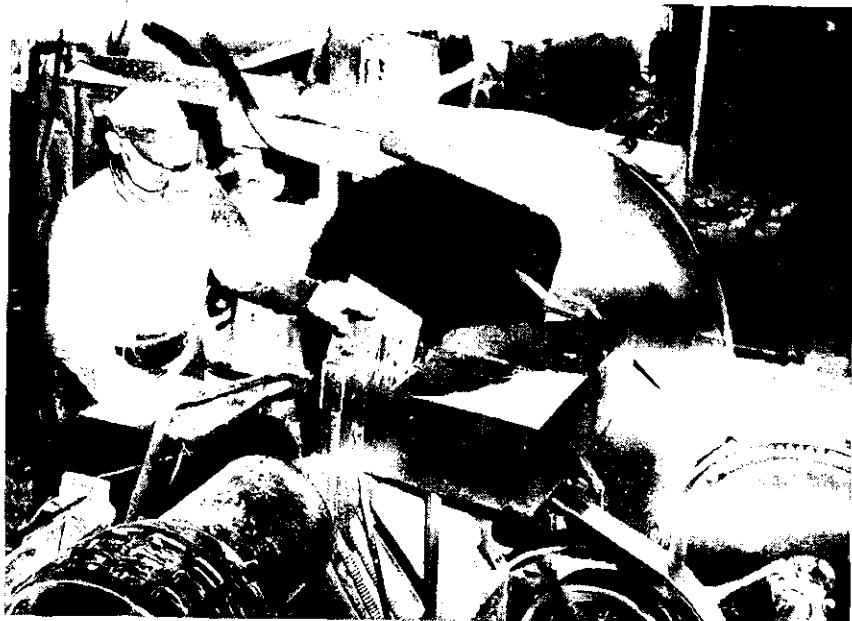
FIG. 10-2. Shingle sawyer trimming edge of a shingle with his right hand as he takes the next shingle from the saw with his left hand. (Courtesy Red Cedar Shingle Bureau.)
