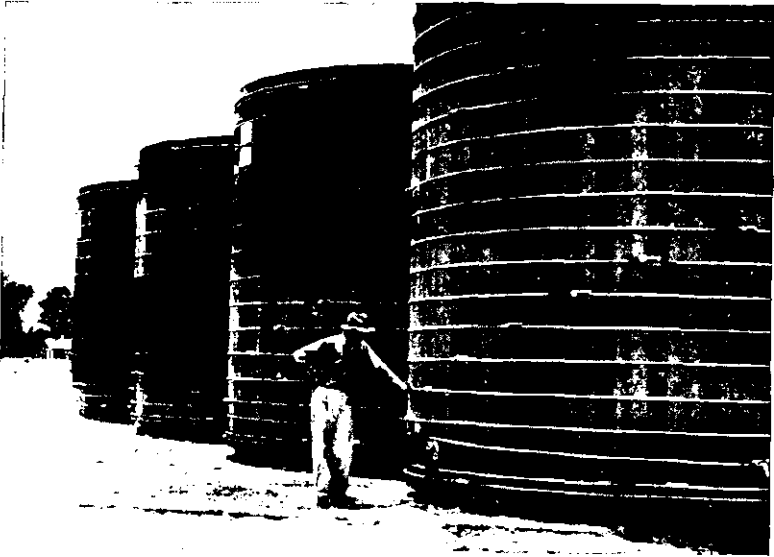
FIG. 9 11. Battery of redwood tanks used for storage of corrosive sour-oil crudes. (Courtesy California Redwood Association.)
