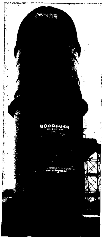
FIG. 2-4. Refuse burner of the Great Southern Lumber Co., Bogalusa, Louisiana. The use of this burner was discontinued in 1924, through utilization of the sawmill refuse in the manufacture of paper. The inscription on the burner reads "Bogalusa Plant of Great Southern Lumber Co. Refuse Burner Born October 1, 1908 Died July 4, 1924. Every day during my life of sixteen years I consumed daily 560 cords of waste material or a total of 2,688,000 cords. I cost $75,000, but my fire has destroyed $1,344,000 worth of what was formerly considered waste. The complete utilization of the sawmill refuse in the manufacture of paper has my fire forever extinguished."
