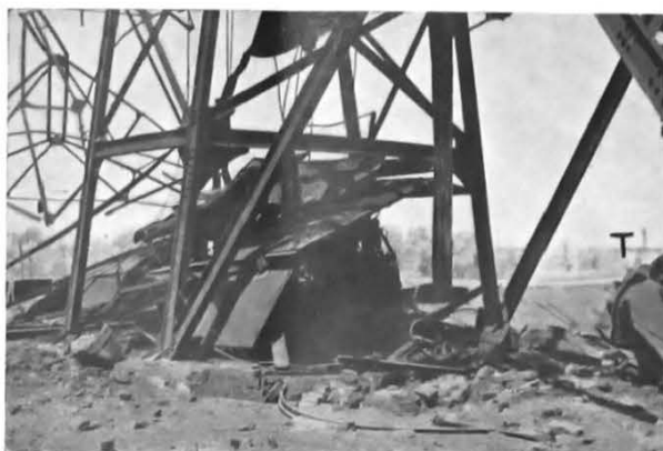
View of upcast shaft after explosions. T. A tub blown up the shaft.
