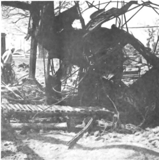
Close up view of wreckage at top of upcast shaft.
