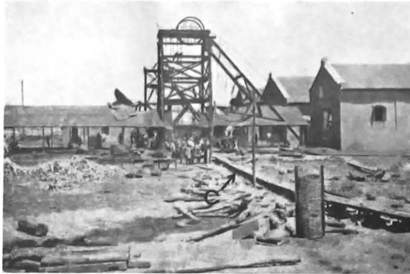
General view with downcast shaft in foreground and conveyor. C. which was used for conveying earth to seal the bottom of the shaft.
