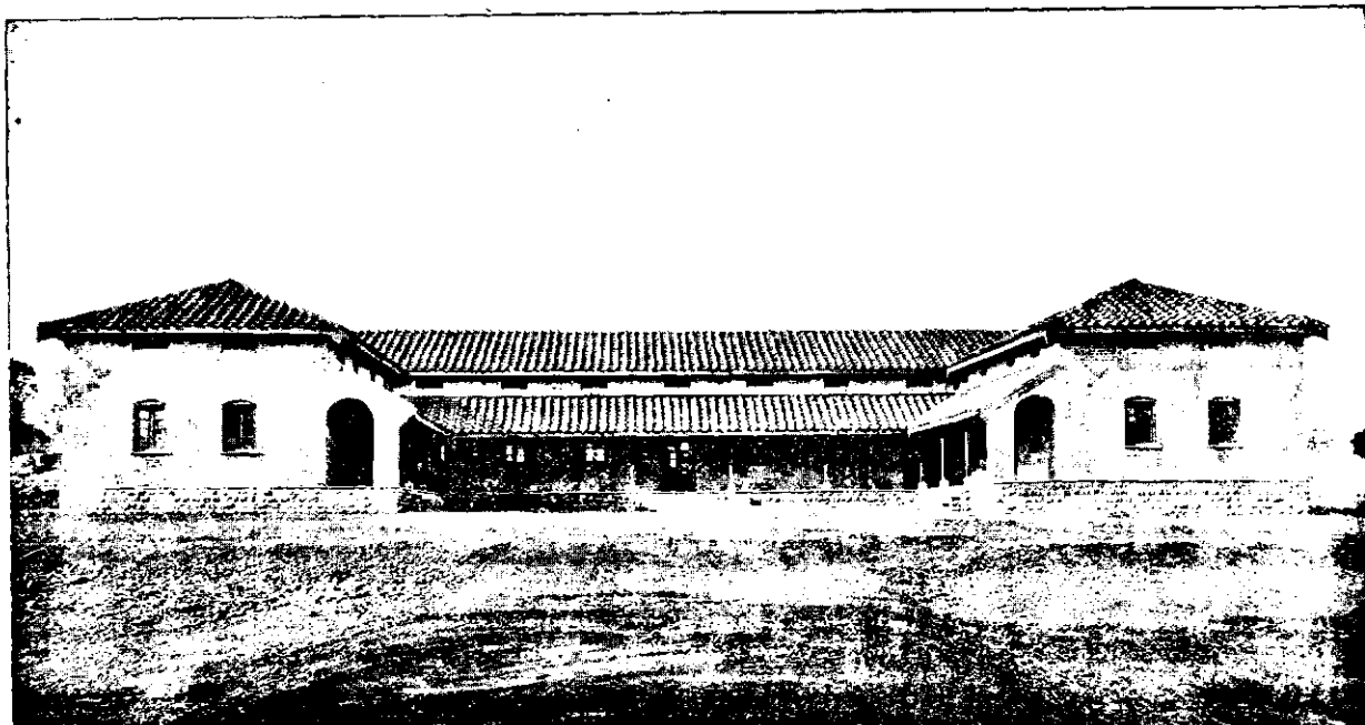
MUNICIPAL PRIMARY SCHOOL, YEOTMAL, CENTRAL PROVINCES.
