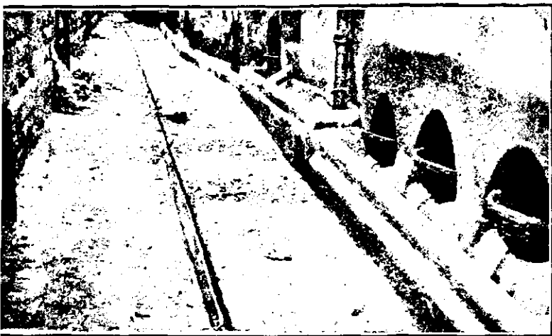
SWEEPER'S GULLY WITH BASKET PRIVIES AND OPEN DRAINS.
