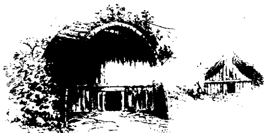
25.—ANCIENT TYPE OF DWELLINGS DISCOVERED IN THE HIMÂLAYAS, AND IN A NUMBER OF PLACES.
