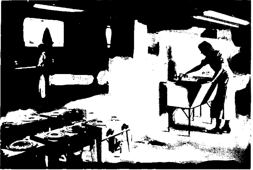
Light, airy, sanitary community laundry in a PWA Housing Division development: Techwood Homes, managed by the Atlanta Housing Authority under lease agreement with the USHA.
