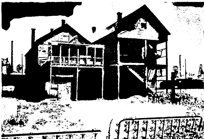
Chicago: Four families live in these two houses—seven people on the top floor of the house at the left. Note the broken steps: From these houses and others like them, as well as from Trumbull Park Homes (see next picture) come workers for neighboring factories.
