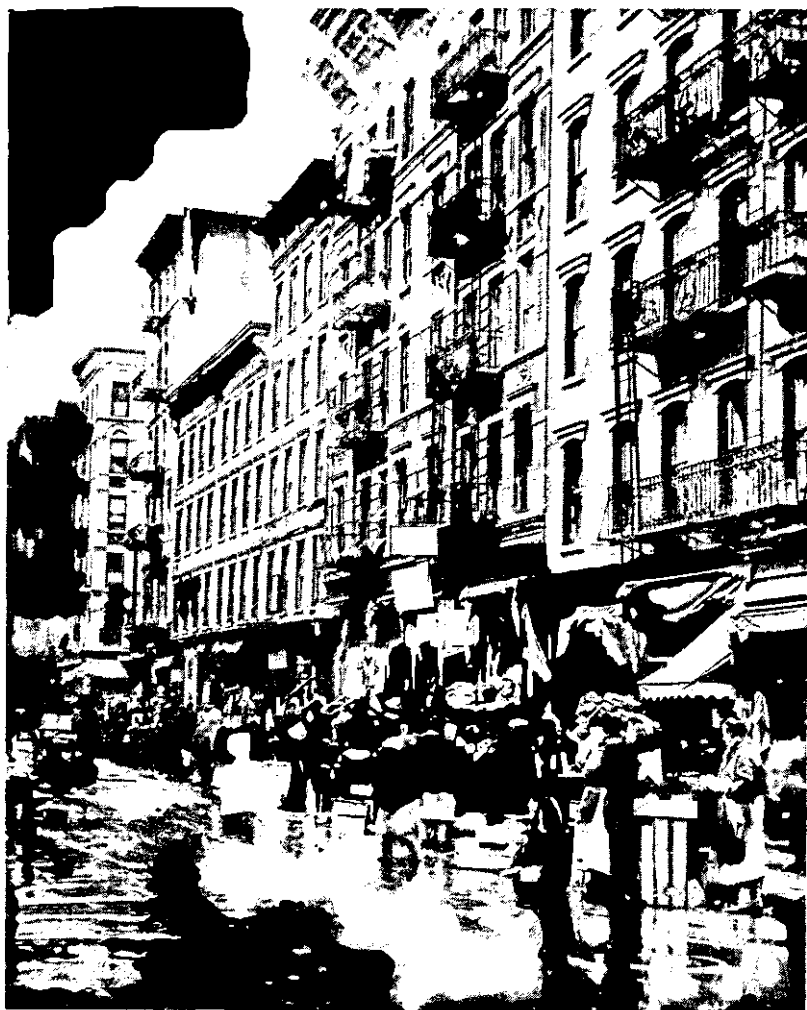
Typical New York City street of old-law tenements: The buildings cover as much as 90 percent of the lots. Many rooms are entirely windowless.
