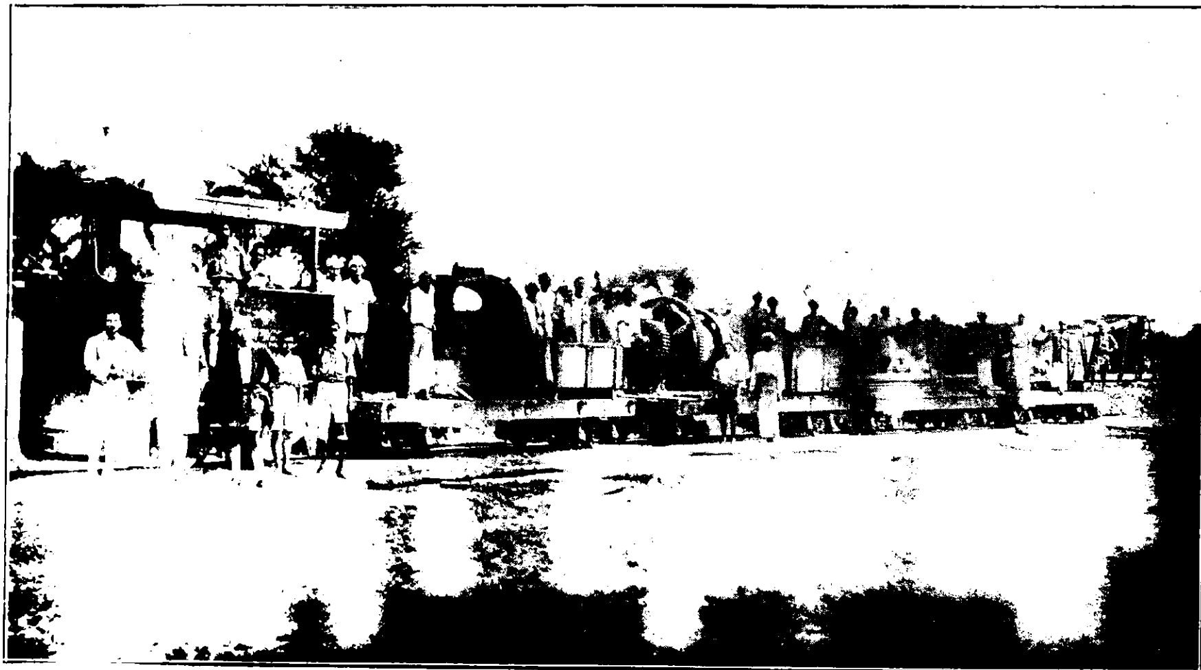
(5) QUARRY (METTUR) PROJECT—SENTINEL WITH BOGIE WAGGONS CONVEYING PARTS OF DRAG LINE EXCAVATOR
