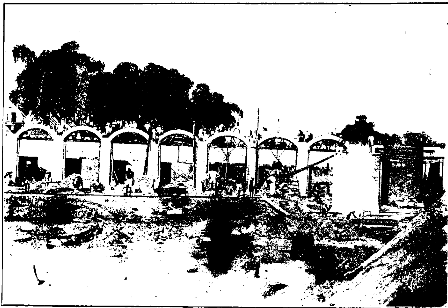
(2) BANDAR CANAL—LOCK AND REGULATOR UNDER CONSTRUCTION
