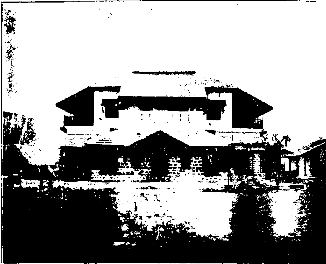
(4) CAUVERY (METTUR) PROJECT - METTUR CAMP - EXECUTIVE ENGINEER'S TYPE QUARTERS
