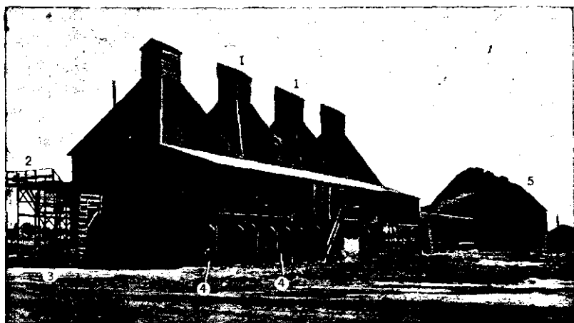
FIG. 290. A typical hop dryer showing ventilating cupolas (1), unloading platform (2), portable derrick platform used in training the vines in the field (3), furnaces (4); and (5) cooling house.
