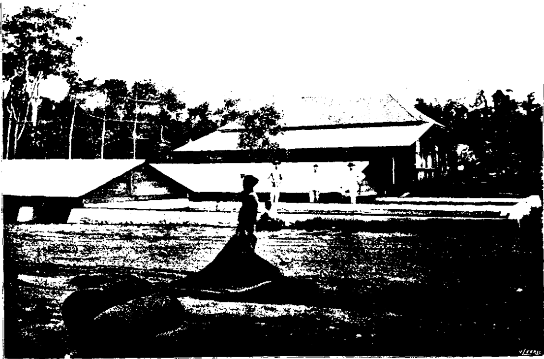
JAVA. STONE COFFEE DRYING FLOORS WITH MOVEABLE ROOFS
