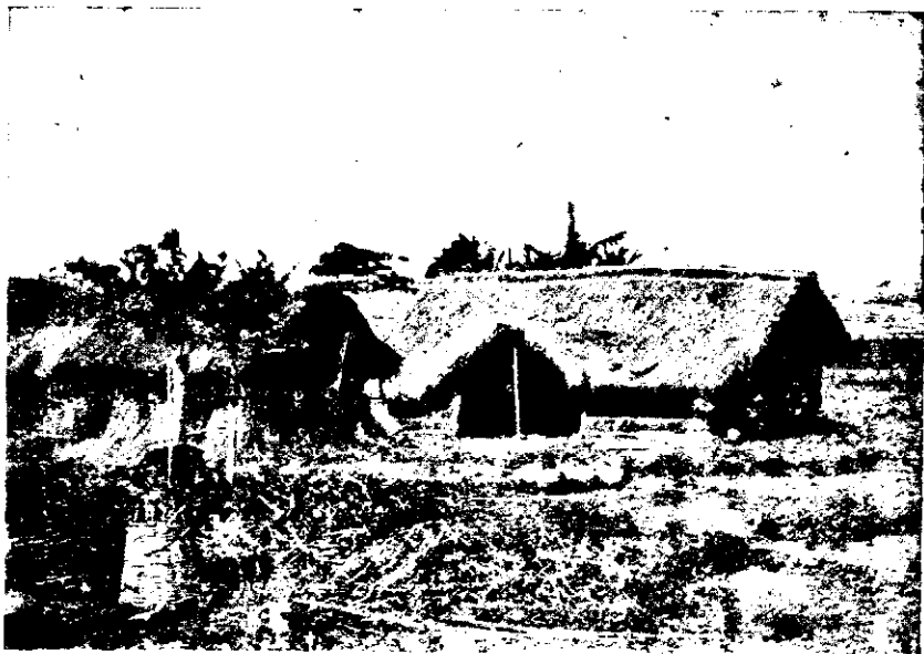
Figure 3. Housing conditions. In the foreground an old type basha. In the middle distance a new house similar in construction to the old one, but larger. In the background the frame-work of a new house.
