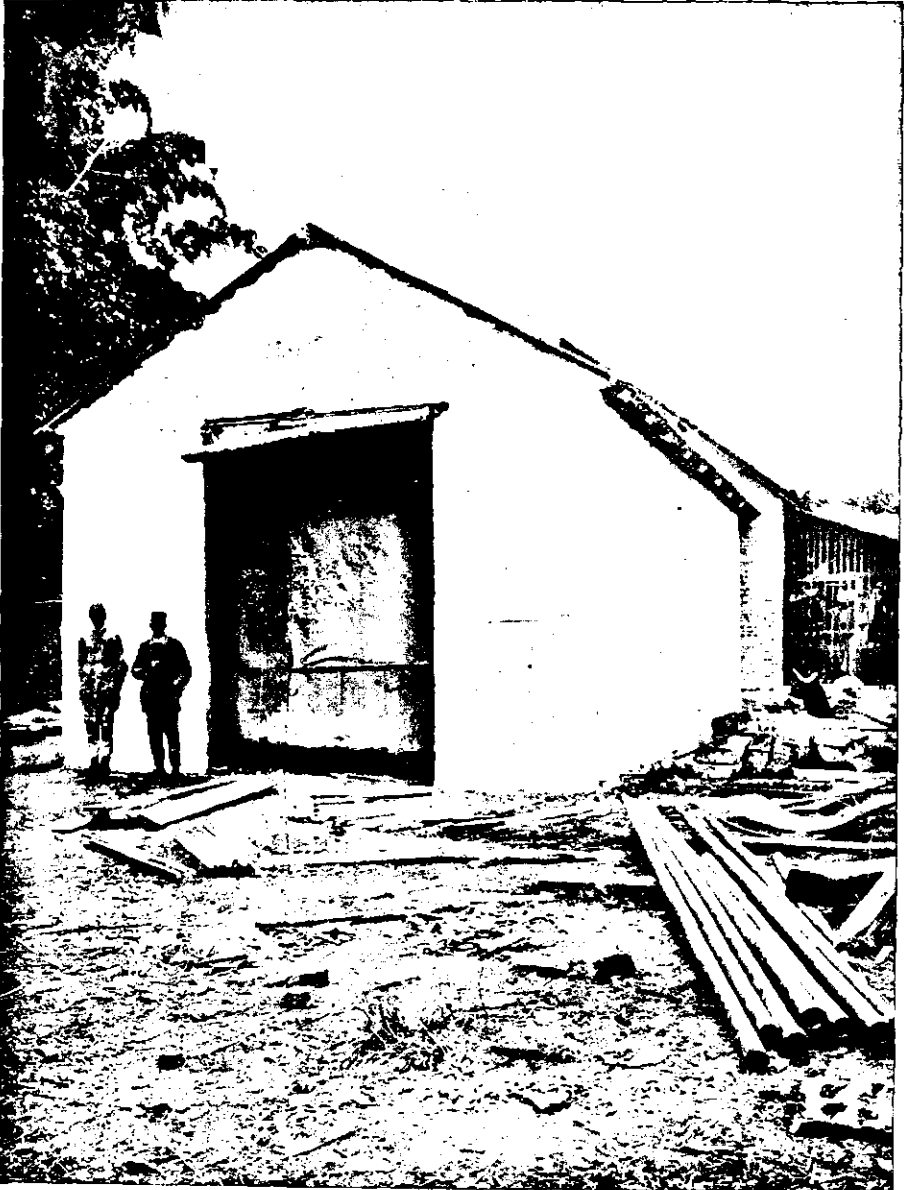
Photo I. A kiln similar to the above has a capacity of approximately 8 tons of box shooks or 2 tons output per day, and may be built for Rs. 5,000 exclusive of the power plant. Its greatest usefulness is probably in connection with small semi-portable saw mills operating in the jungle.
