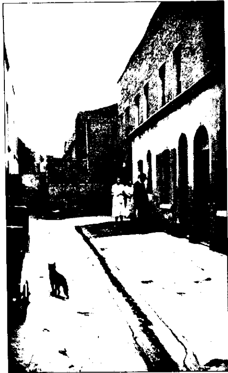
Another court with open drainage channel in the centre.
