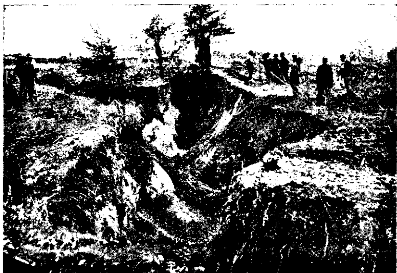
FIG. 123. —Gully head in North Carolina. Dynamite was used for sloping the sides of this large gully. Holes for the charges are being dug. (Courtesy of U. S. Soil Conservation Service, North Carolina.)
