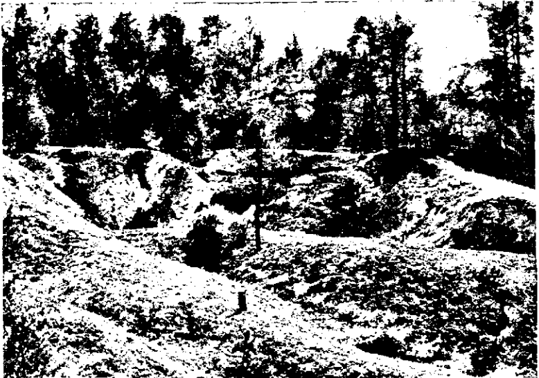
FIG. 120. —Gully treatment in North Carolina. II. Comparative treatment of a vegetative nature is in progress. Locusts, pines, and lespedeza have been planted and the surface mulched with pine forest litter. These gullies must be stopped before they ruin more good land.
