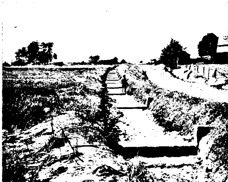
FIG. 90.—Old highway developed into a terrace outlet. This satisfactory terrace outlet has a slope of 7 per cent. Note the protection afforded by the concrete baffles. The workers on this Soil Conservation Service project at Spartanburg, S. C., feel that this outlet could be protected with sod.
