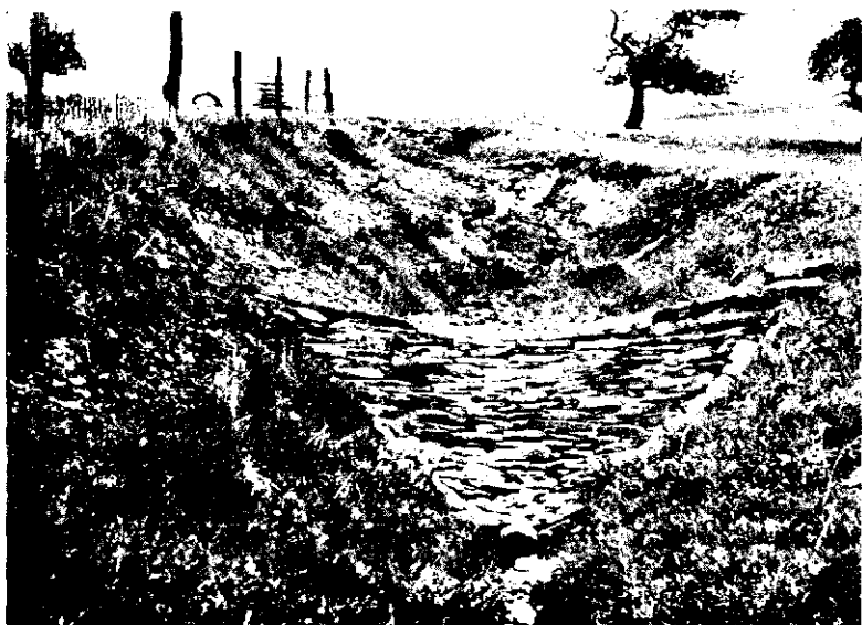
FIG. 80.—Diversion-ditch outlet. This moderately well stabilized gully serves as outlet for the ditch shown in Fig. 79. Honeysuckle (bush type) is planted on the raw banks near the stone dams. In southern New York.
