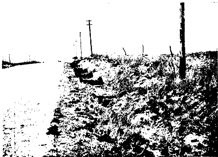
FIG. 177.—Creosoted plank check dams in central Illinois. Slope of road ditch 6 per cent. Data supplied by T. R. Wire of the U. S. Demonstration project at Le Roy, Ill.
