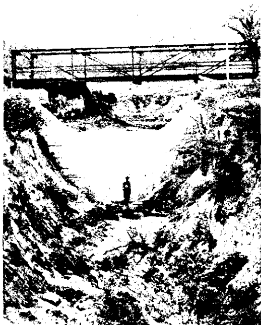
FIG. 136.--Concrete soil-saving dam. The underlying soil material here erodes with extreme ease. The following year this dam washed out and fell over into the gully. Photographed by the writer in Mason County, Illinois, 1912.
