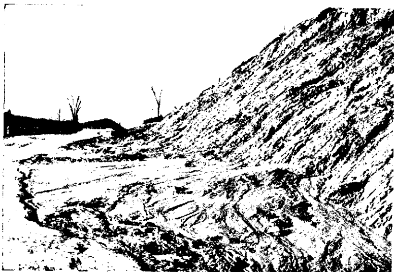
FIG. 173.—Lake-laid soil in New York, unstable when wet.
