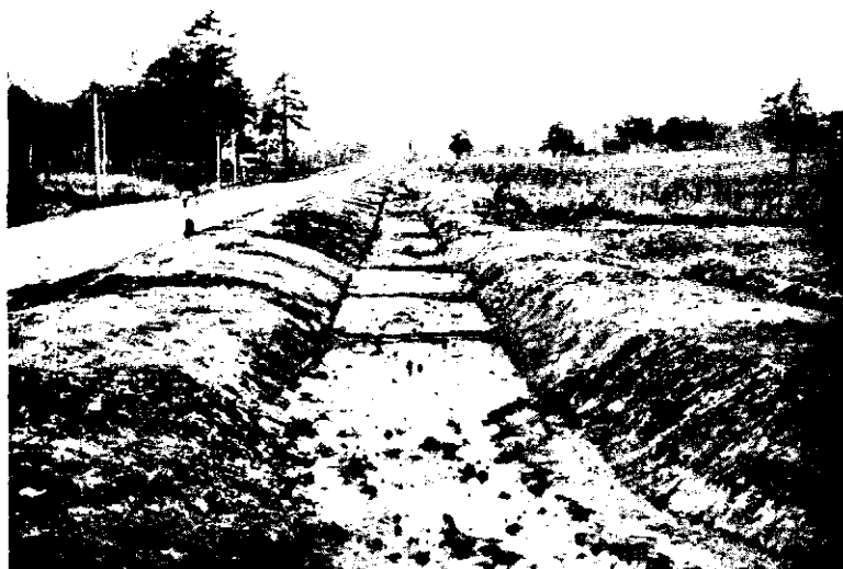
FIG. 86. Terrace outlet in North Carolina. The baffles have been constructed and the bottom and sides are ready for seeding. (Courtesy of U. S. Soil Conservation Service, North Carolina.)
