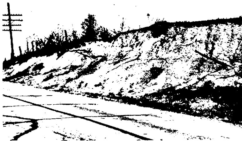
FIG. 175.—A slip on a road cut in southern Ohio.
