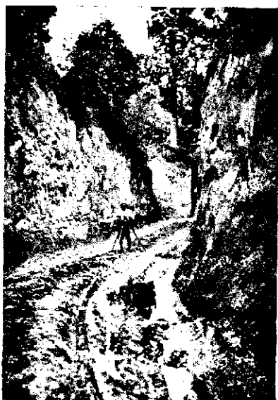
FIG. 172.—A road in a depression in deep loess. Erosion has lowered this roadway. No outlet for water is possible, except down the highway. Photographed in western Illinois, 1912.
