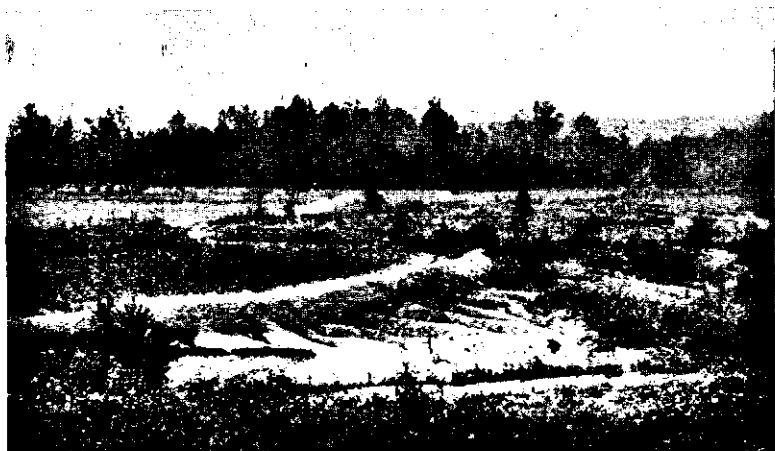
FIG. 111.—Diversion ditch to stop gullying. This ditch diverts the water which collects on the slope above and conducts it to a safe place of disposal in the forested area in the background. In North Carolina, lespedeza seeded under a light protection of straw or pine needles soon reclothes an area such as this with protecting vegetation. (Courtesy of U. S. Soil Conservation Service, North Carolina.)
