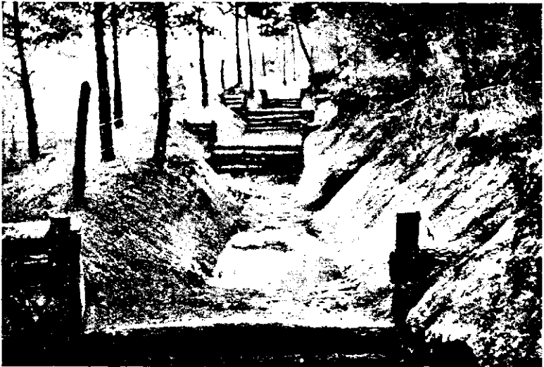
FIG. 92.— Stabilized gully serving as terrace outlet. This gully was stabilized by means of log check dams. The use of vegetation in addition will be helpful. This is the same gully as shown in Fig. 91. (Courtesy of U. S. Soil Conservation Service, North Carolina.)
