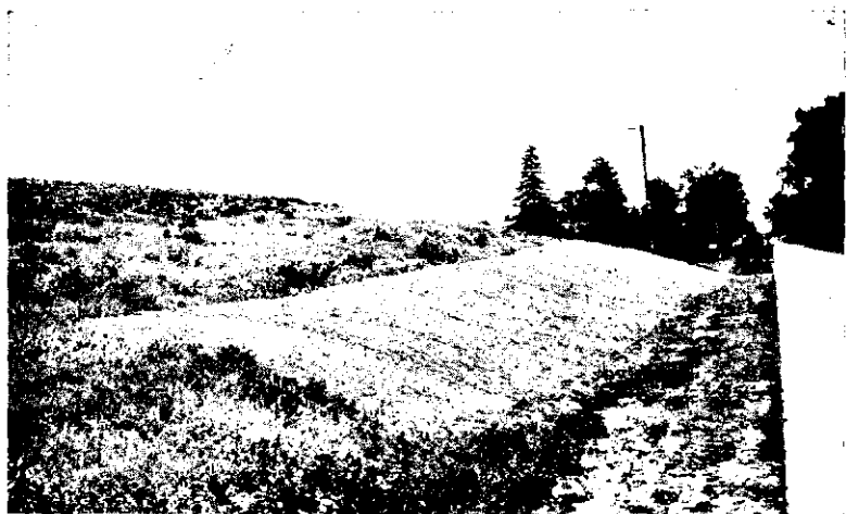
FIG. 186.—Newly seeded well-sloped cut. This cut has been sloped to approximately 33 per cent. The soil is dry. When the grass becomes established, erosion on this cut will be under control.
