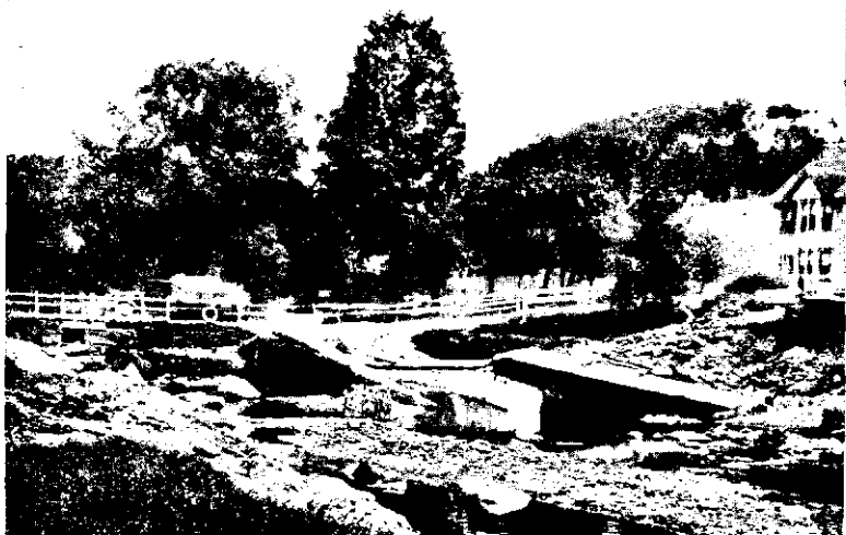
FIG. 190.—Flood damage to a state highway bridge. A few hours before the prolonged rains of July 7 and 8, 1935, this was a good concrete highway bridge in Delaware County, New York.
