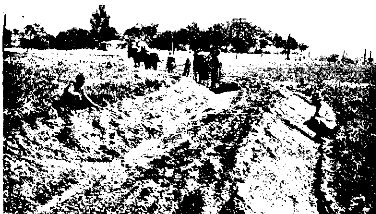
FIG. 95.—Farmer-constructed terrace. This terrace, on the J. M. Dean farm three miles west of Spartanburg, was constructed with two-horse, No. 13 Oliver plow with extension moldboard and homemade, V-drag. Six rounds were made in the construction. Width of terrace, 12 feet, height 18 inches. Back furrowing had not been done when photographed. (Courtesy of U. S. Soil Conservation Service, Spartanburg, South Carolina.)
