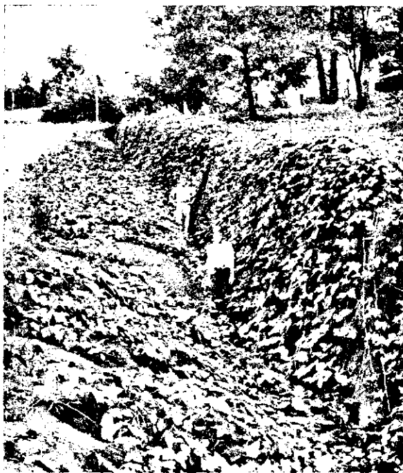
FIG. 182.—Kudzu controls erosion in highway ditch, in South Carolina. Note how completely the kudzu vines cover the soil. A wide extension of the planting of kudzu in ditches and gullies in the South is highly desirable. (Courtesy of U. S. Soil Conservation Service, South Carolina.)
