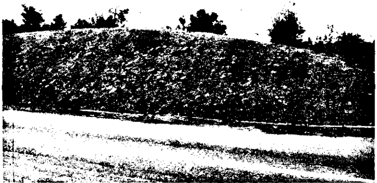
FIG. 185.— Recently sodded road cut. This road cut in western New York was covered with turf. Slope between 50 and 60 per cent. Such treatment affords excellent protection on well drained soils.
