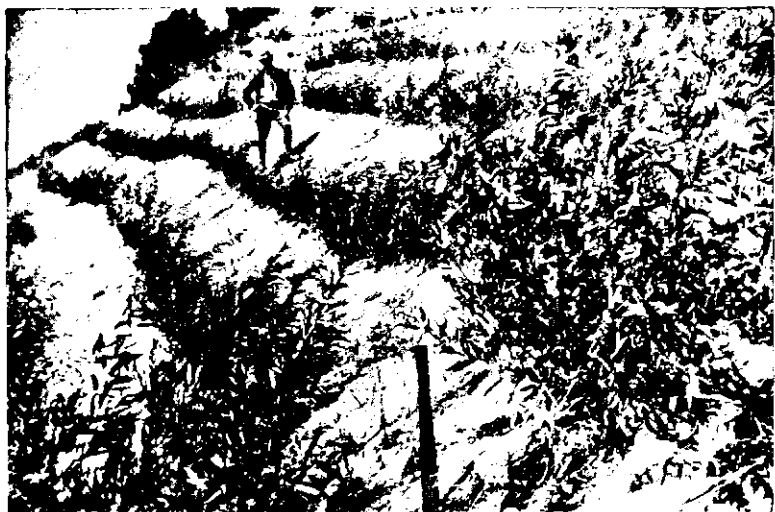
FIG. 189.—Wattle and stake growth on a steep slope in California. This growth was made in 6 months from stakes of common red willow ( Salix laevigata ) set to hold wattles in place. (Courtesy of C. J. Kraebel, California For. Exp. Sta., U. S. Forest Service.)
