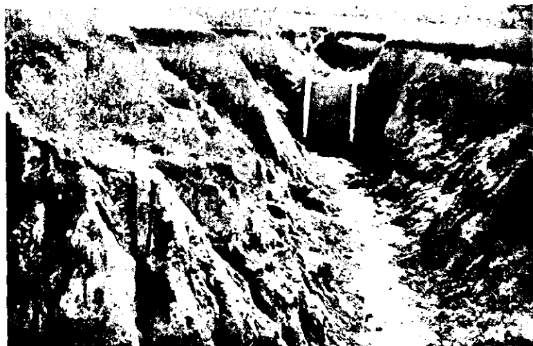
FIG. 137. Concrete check dam. In soils underlaid by incoherent sand it is almost impossible to extend the ends of dams into the solid sides far enough to make them safe. The apron has already been undercut. Vegetation may be of real value in gullies of this nature. Photographed, Illinois, 1913.
