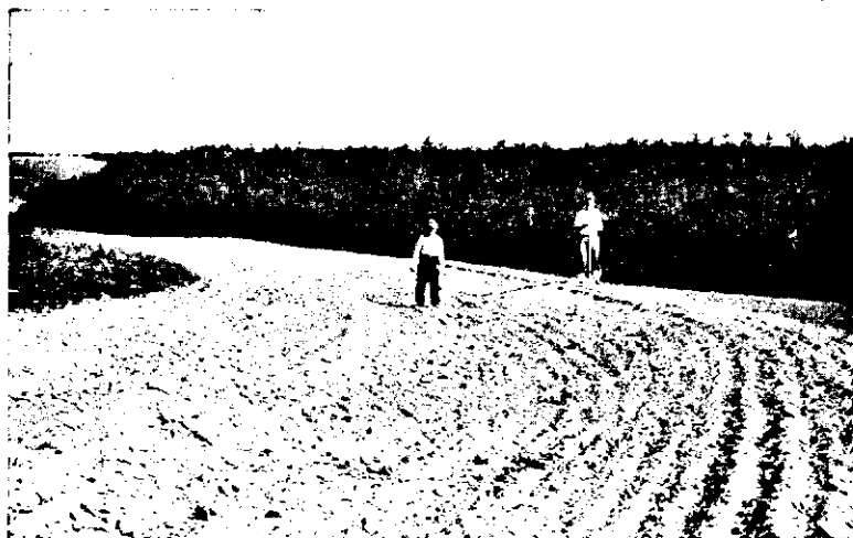
FIG. 78.—Diversion terrace in New York. This diversion channel is 8 feet wide and 17 inches deep with a fall of approximately 12 inches in 100 feet or 1 per cent. This ditch is expected to carry the water from 12.5 acres of land with a slope of 6 per cent immediately above the channel. This is in every sense a Nichols terrace. Details supplied by N. J. Curtis.
