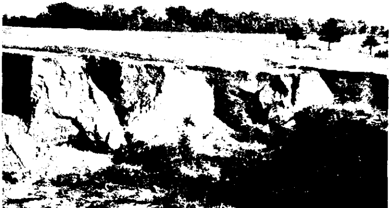
FIG. 93. Gully traceable to road drainage. The cause of this gully appears to have been drainage water from the highway. Each notch on the other side of the gully is the end of a terrace water channel. A well-protected terrace outlet parallel to the big gully is needed. Near Spartanburg, S. C.
