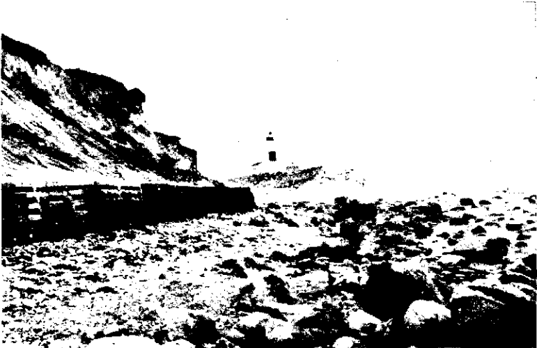
FIG. 156.—Erosion on the Atlantic Coast of Long Island. This rock pavement or barrier is insufficient to protect the coastline which is composed of glacial materials. Erosion of glacial soil materials is unusually rapid.
