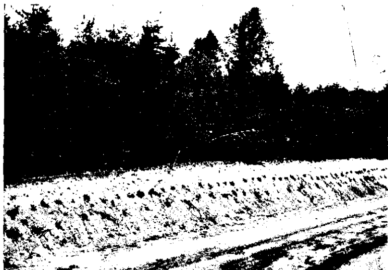
FIG. 179.—Road-cut planting in Virginia. This planting included the trumpet creeper ( Tecoma radicans ), dewberry ( Rubus villosus ), myrtle or common periwinkle ( Vinca Minor ), and black locust ( Robinia Pseudo-acacia ).
