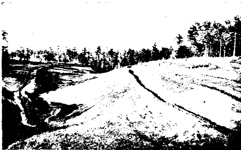
FIG. 126.—Darby-High gully treatment in South Carolina. This gully had cut back and caused the moving of the public highway to its third location. The sides were cut down, diversion ditches made for conducting the road water into wooded area at the right. Bands of Bermuda-grass sod were placed in the ditch. Small grain was seeded and black locusts were planted 4 feet apart. (Courtesy of U. S. Soil Conservation Service, Spartanburg, South Carolina.)
