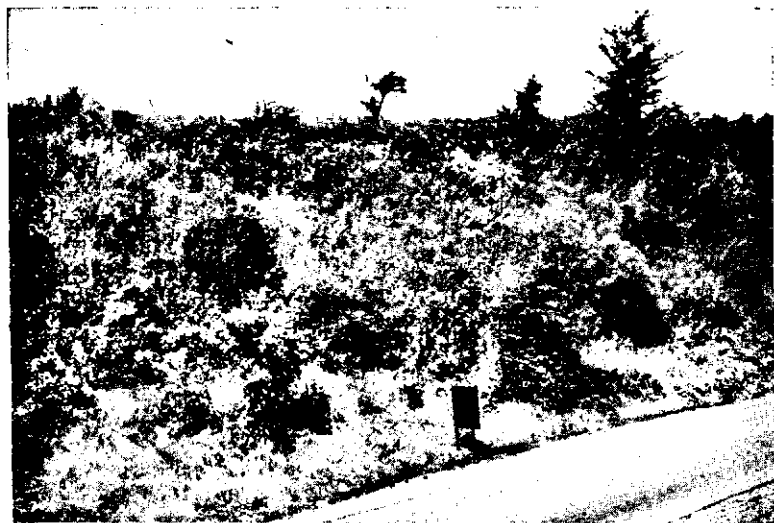
FIG. 187.—Nature protects a road cut in central New York. Nature needs assistance, however, in order to eliminate erosion quickly. The following plants were found in this natural roadside protection:
