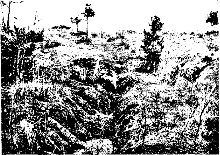
FIG. 129. Gully treatment with brush. I. Note the sediment caught and held by the brush. (Courtesy of U. S. Soil Conservation Service, North Carolina.)
