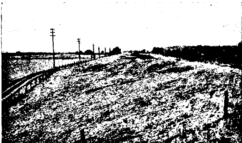
FIG. 195.—Levee protecting farm land along the Illinois River. Note the willows on the river side of the levee. Keeping these down permits the water to get away and reduces the crest of floods locally. But while doing this it hastens the attainment of and raises the crest of floods on the Mississippi.
