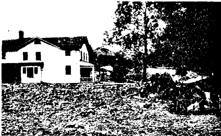
FIG. 193.—Flood damage to a suburban home. This lawn is covered with stones to a depth of several feet. The roof of an automobile has been uncovered at the right. The flood water had covered it completely.
