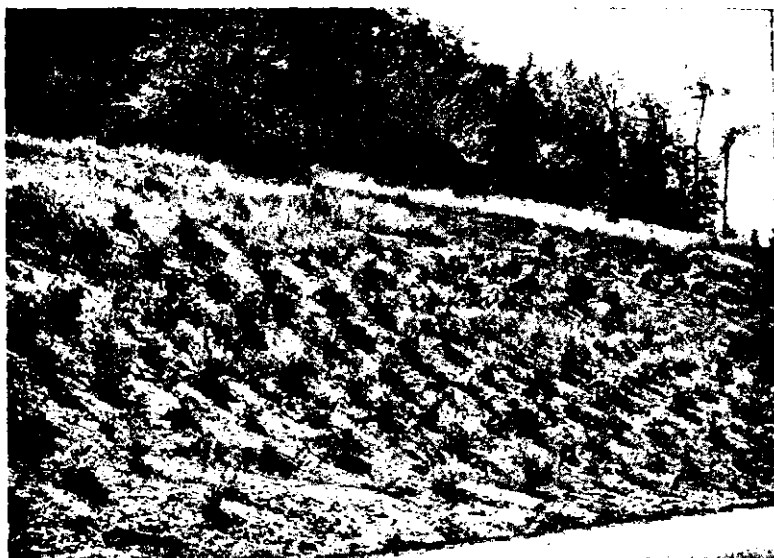
FIG. 184a.—Shrubs on left side of road in central New York. Figure 184a is directly opposite Fig. 184b. The slope varies from 40 to 60 per cent. Virginia creeper is planted nearest the roadway. It is very fitting to plant shrubs on this side since they blend with the adjacent trees.
