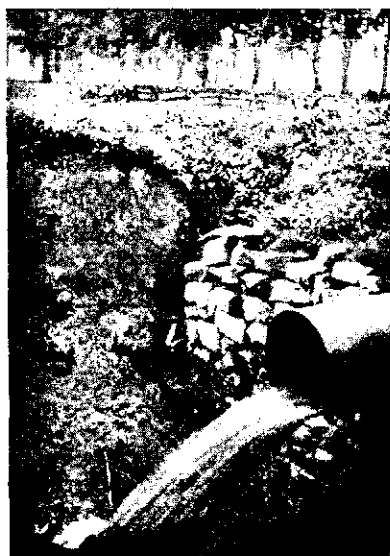
FIG. 171.—Discharge of water by a steel road pipe. If this water does not fall on rocks, brush, concrete, or other stable material undercutting of the road is inevitable. Photographed in central Illinois in 1914 following a shower.
