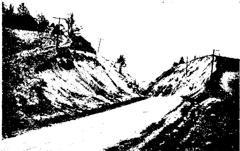
FIG. 165.—A highway cut in eastern Tennessee. Some of this cut is through rock but soil has rolled down over it.
