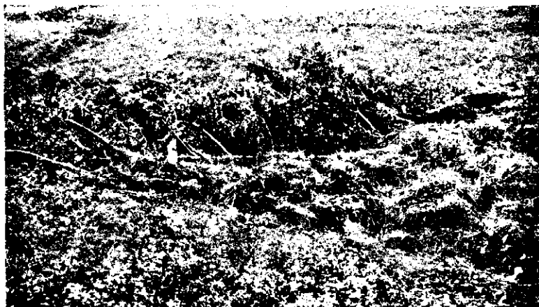
FIG. 133. - Brush dam completed. III. The dam has been completed and the wet straw placed for catching the silt washed from the fields above. (Courtesy of Ivan D. Wood, Nebraska Agr. Ext. Service.)
