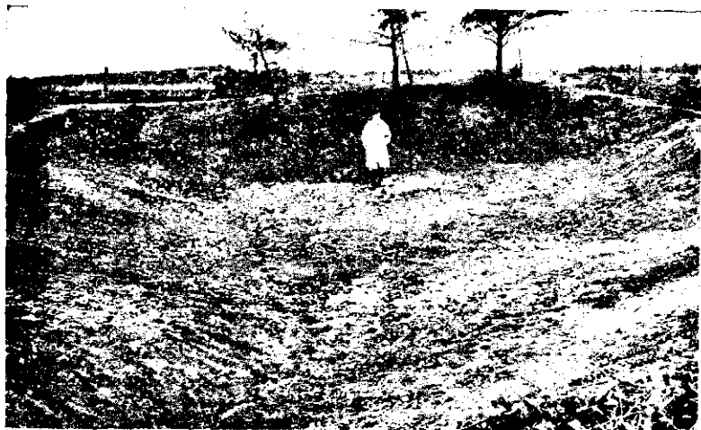
FIG. 124. Completed gully sloping. The gully shown in Fig. 123 after sloping treatment. The slope on the sides was reduced to 3 to 1, or 33 per cent. March 11, 1936. This gully is ready for seeding and mulching. Lespedeza and locusts could be very helpful in a situation such as this. (Courtesy of U. S. Soil Conservation Service, North Carolina.)
