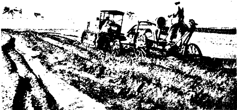
FIG. 94.—Terracing in Oklahoma. This broad-base terrace is being built with heavy terracing machinery. A few more rounds complete the ridge. (Courtesy of U. S. Soil Conservation Service, Oklahoma.)
