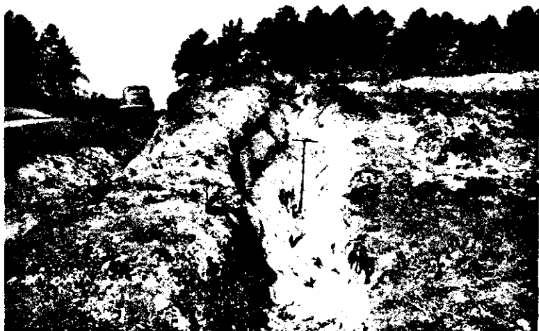
FIG. 176.—Road-cut diversion ditch. The road-cut diversion ditch is a good device. In this case water from a field road was turned into it. The additional water caused this erosion. Slope about 12 per cent. Photographed in North Carolina.
