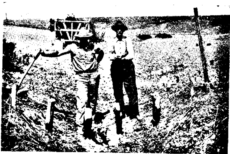
FIG. 131.—Building a brush dam. I. The posts are in place for the one-row post brush dam. (Courtesy of Ivan D. Wood, Nebraska Agr. Ext. Service.)
