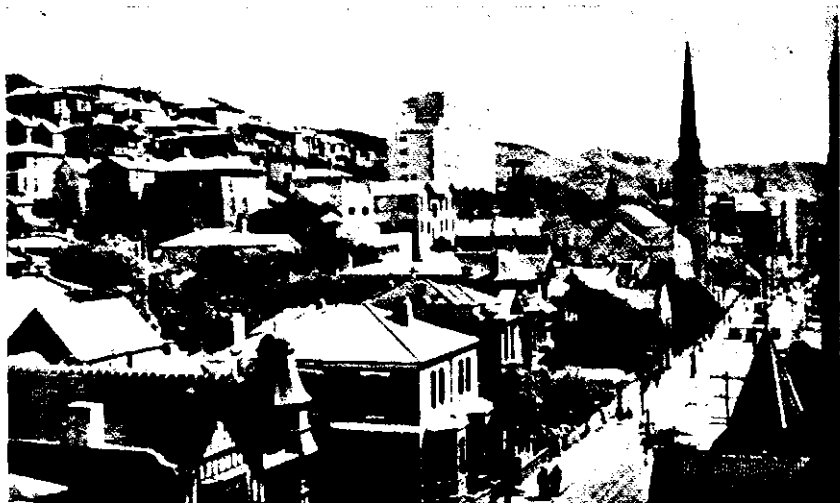
State apartment house projects (rear center) in Wellington, New Zealand, initiated by Labor government. (Courtesy New Zealand Legation)
