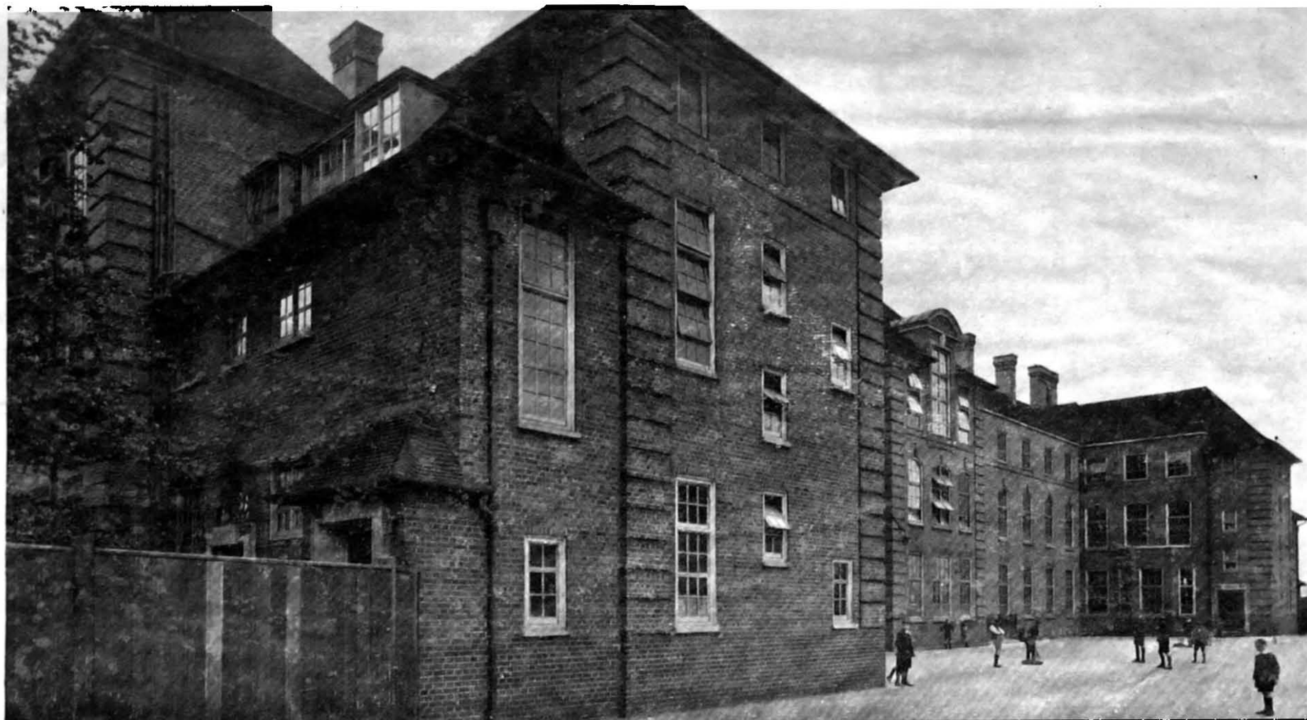
HILLBROOK ROAD ELEMENTARY SCHOOL, TOOTING.
