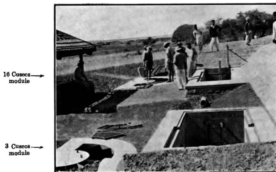
1366.—8 and 16 cusecs Gibb modules (standard design) at the head of Distributary 8, Nira Left Bank Canal.
