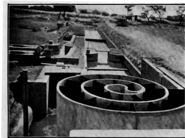
929.—One cusec Spiral module with 3 semi-circles.
