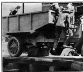
FIG. 11.—Auto-truck box with hopper bottom.
