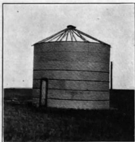
FIG. 13.—Galvanized-iron bin set up in the grain field.
