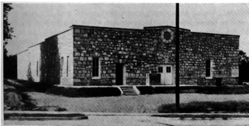
FIGURE 9.—WAREHOUSE AND COLD STORAGE PLANT BRANDON, MISS., LEASED BY THE RANKIN COUNTY COOPERATIVE (A. A. L.)
