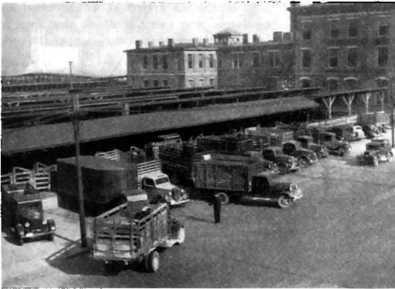
FIGURE 24. ACTIVITIES AT THE TRUCK UNLOADING DOCKS. Hundreds of trucks each day deliver livestock to the Cincinnati Union Stockyards.
