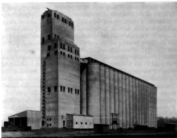
FIGURE 11.—FARMERS NATIONAL GRAIN CORPORATION ELEVATOR AT AMARILLO, TEX.
