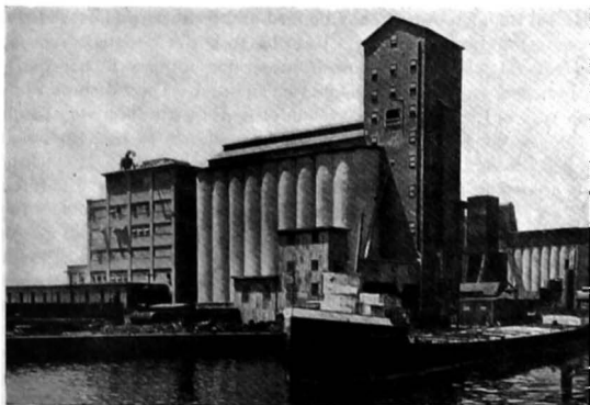
FIGURE 2.—MODERN MILL AND ELEVATOR OF THE GRANGE LEAGUE FEDERATION EXCHANGE, INC., AT BUFFALO, N. Y.
