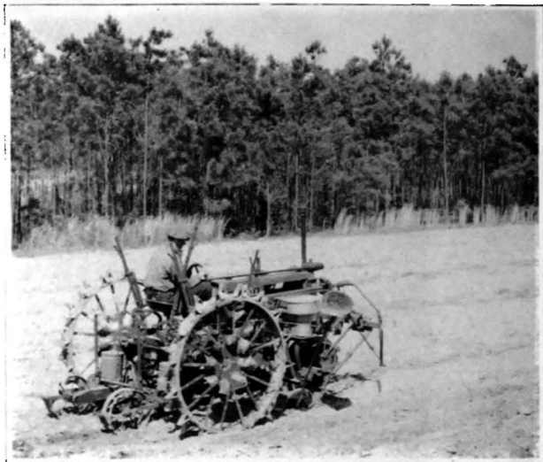
FIGURE 21.— PLANTING COTTON AND PUTTING DOWN FERTILIZER IN ONE OPERATION
