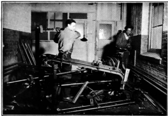
WPA - National Research Project (1936)
