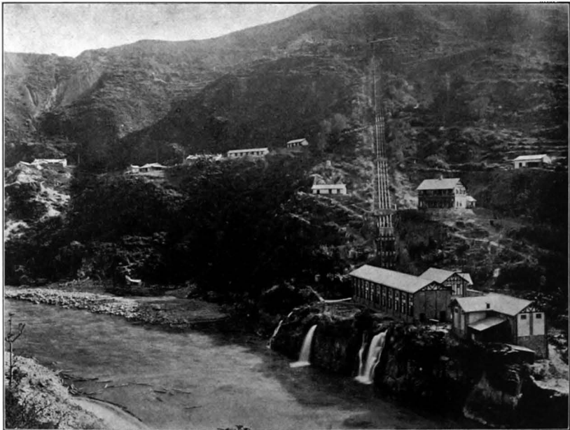
Simla Hydro Electric Works; Power House and Pipe Line.
