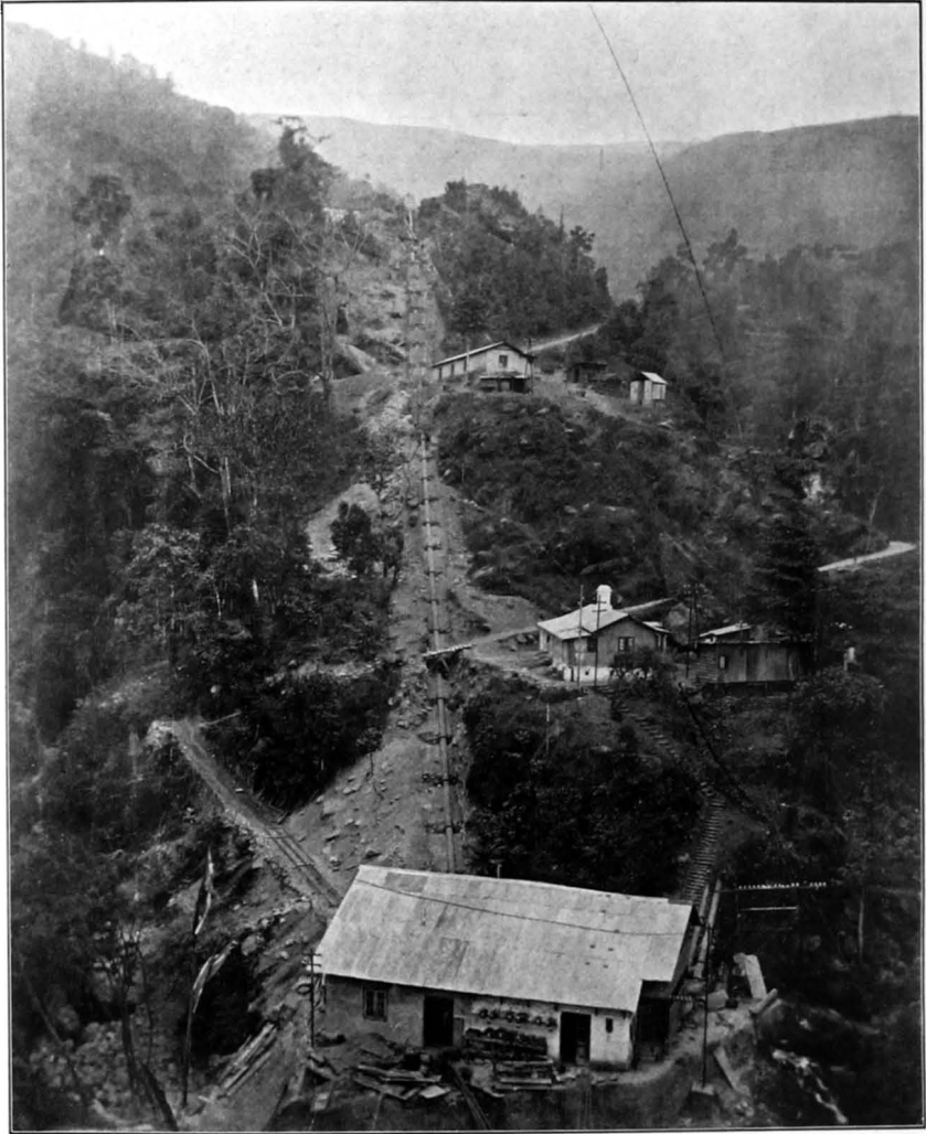
Darjeeling Municipal Electric Works ; the first hydro-electric works in India, erected 1897-8.
