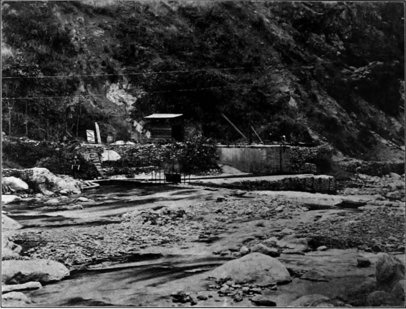
Simla Hydro Electric Works; The Head Works.
