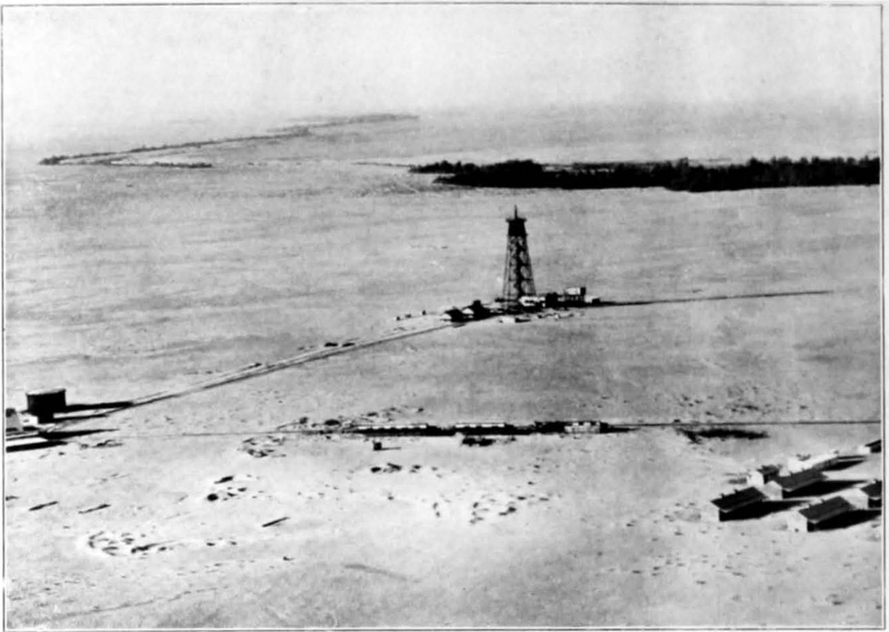
The Intermediate Refuelling Base in course of construction at Ismailia, Egypt.
