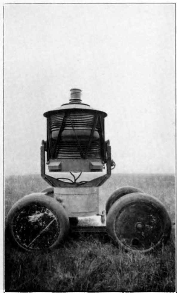
The Portable Floodlight (which is being superseded by a floodlight mounted on a power-driven chassis).
