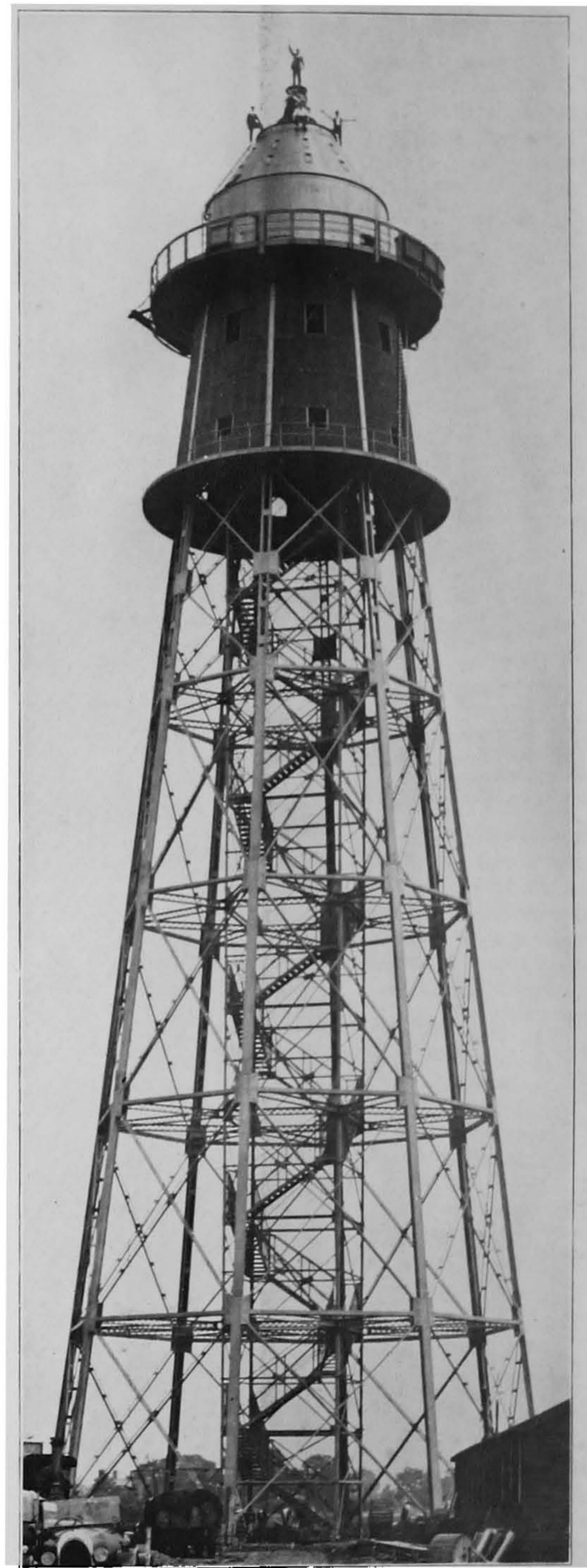
The new Mast at Cardington.
