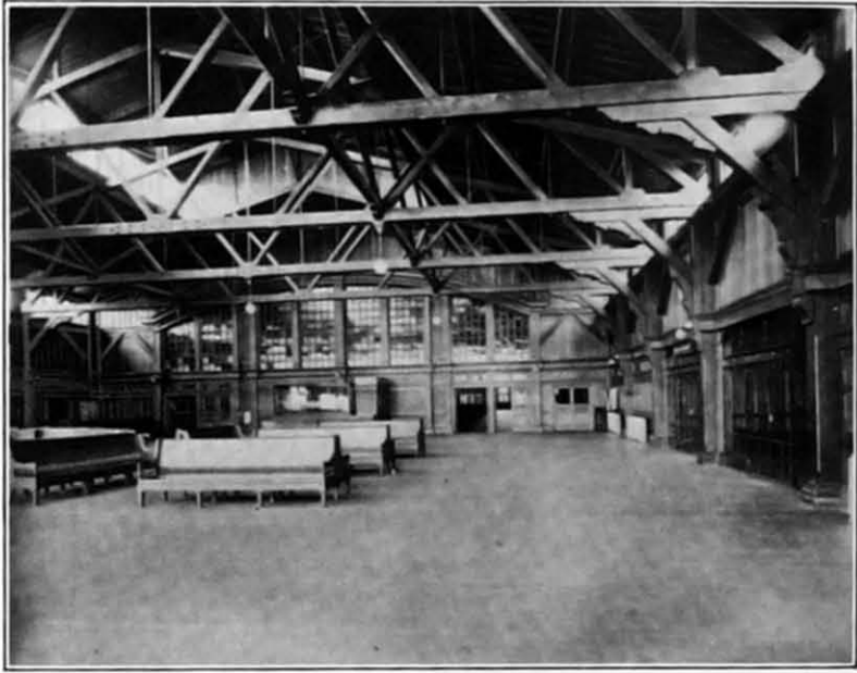
Example of Douglas Fir as structural material in reception room, C.P.R. dock, Vancouver.
