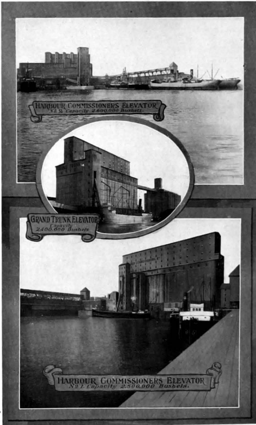
Some of Montreal's great elevators.
