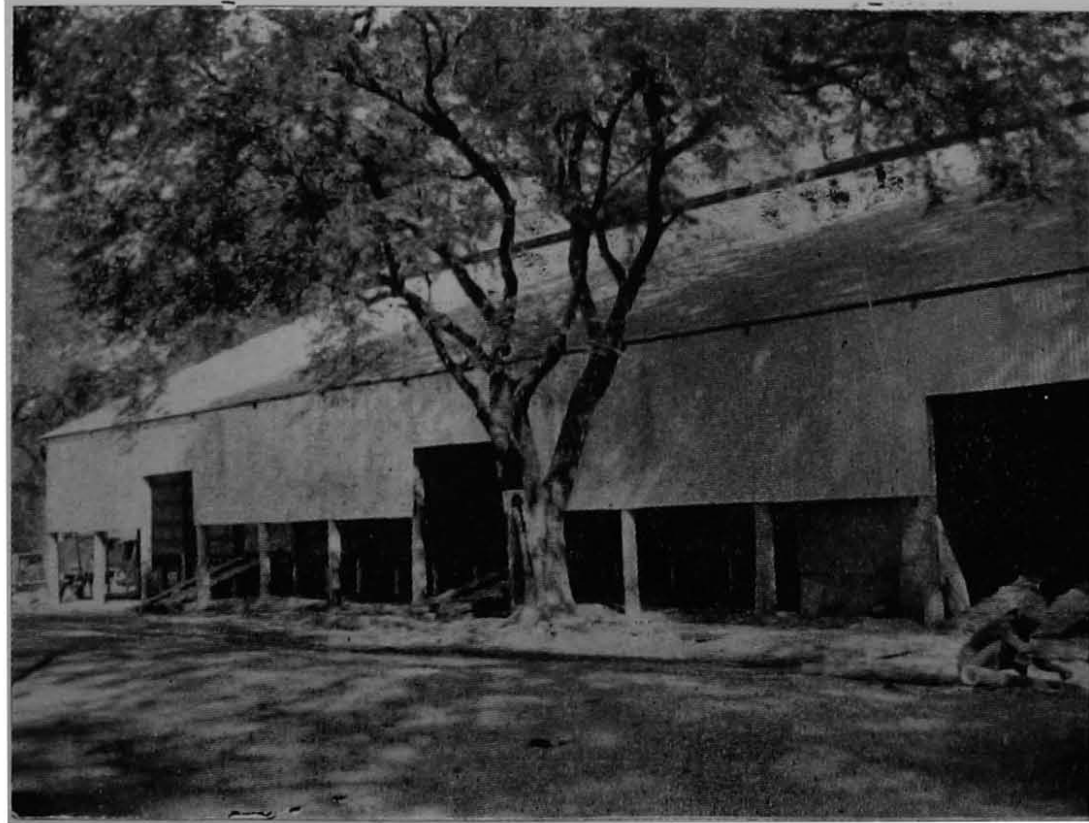
A WELL-DESIGNED PADDY GODOWN, WITH RAISED FLOORS (BURMA).
