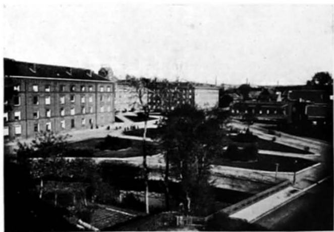
Fig. 4. PRINCIPAL GROUP OF BUILDINGS.
