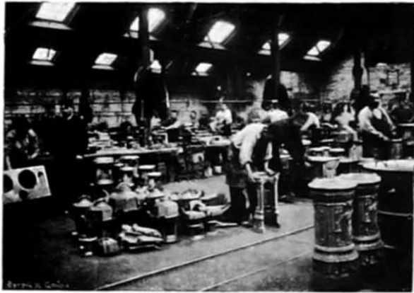
Fig. 39. PART OF THE FITTING-UP SHOPS.
