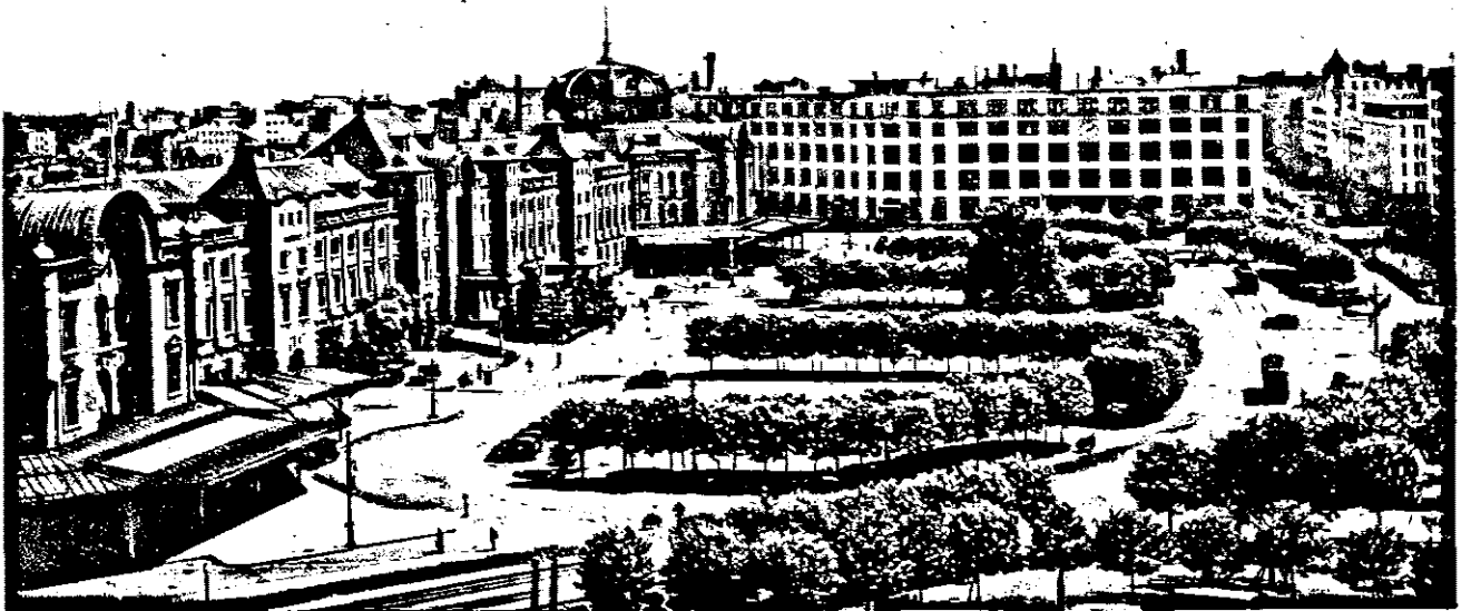
Tokyo Station & Its Vicinity
