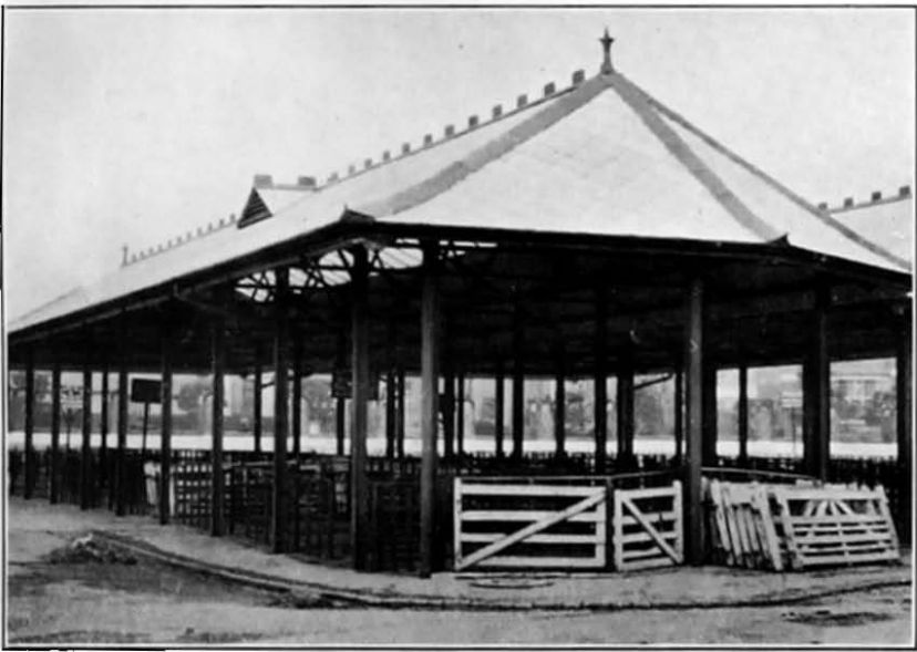
FIG. 20.—Covered pig pens at Peterborough.
