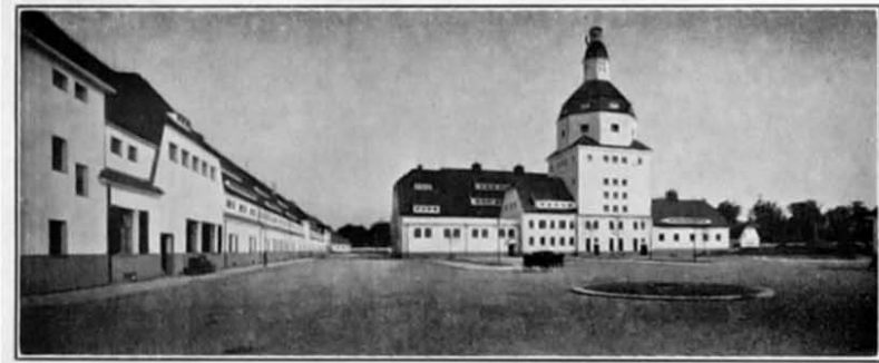
FIG. 32.—Cold Store and Power House.
