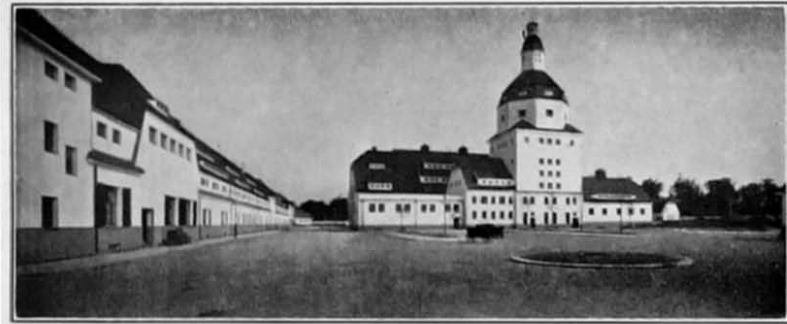
FIG. 32.—Cold Store and Power House.
