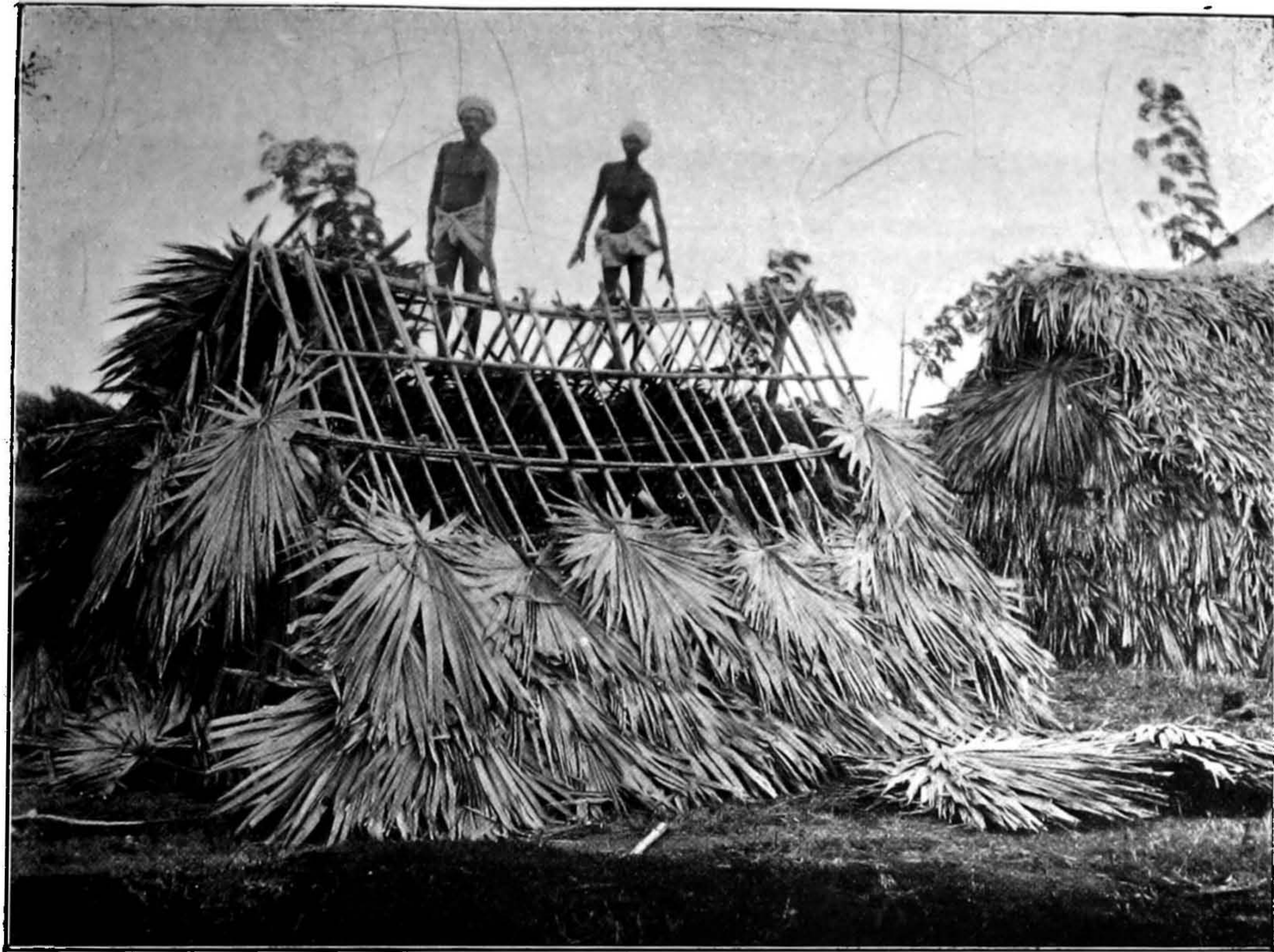
ROOFING A HUT WITH PALMYRA LEAVES.
