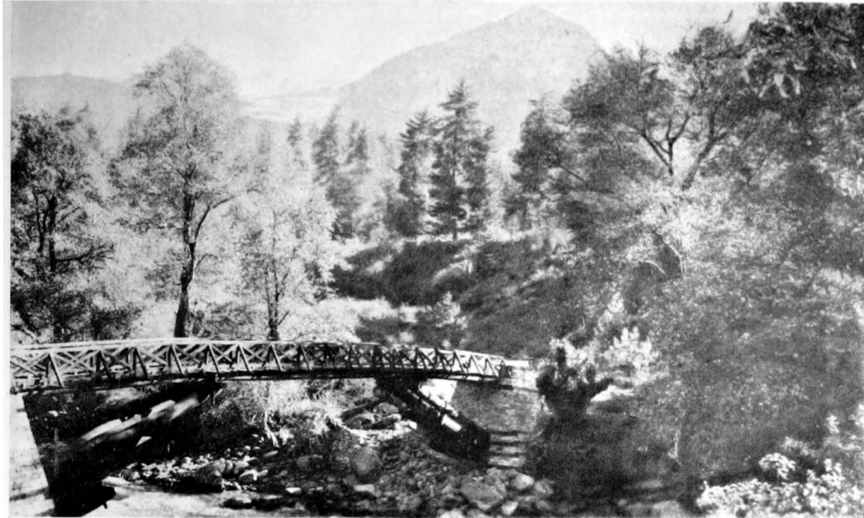
CANTILEVER BRIDGE ACROSS THE BEAS RIVER, KULU, BUILT OUT OF KOTHI FUND MONEY.
