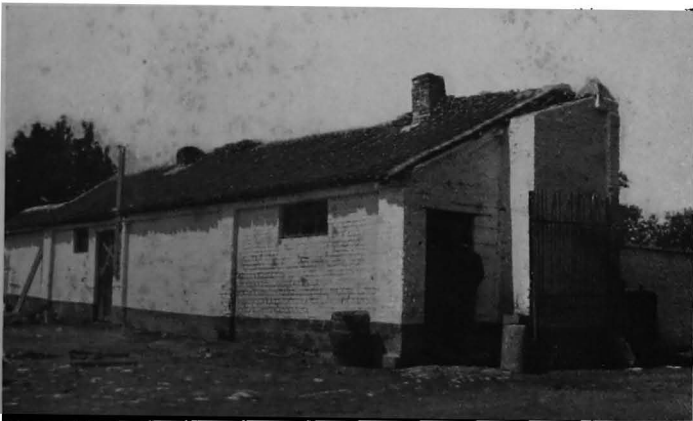
BUILDING USED FOR HOUSING GANG LABOUR
