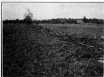
FIG. 87. — Clearing up a fence and brush line so that two fields may be worked together.
