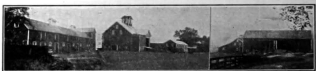
FIG. 99. — Too many buildings for a 190-acre farm, hence they are in poor repair.
