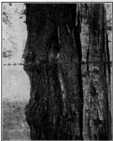
FIG. 95. — A tree makes an unsatisfactory post. The wire spoils the tree and the tree spoils the fence.
