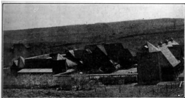
FIG. 100. — A set of barns that cost $600 for each animal housed. At least six times too expensive. Too large for the farm. Poor construction, as the low, many-gabled roofs allow little storage room and are very expensive to maintain.
