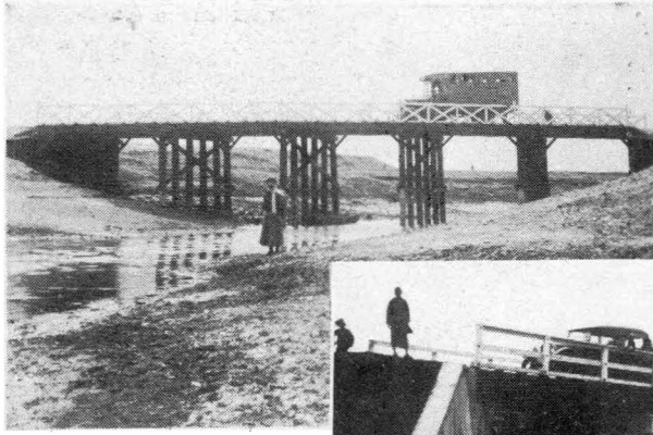
Above—One of the New Timber Bridges —Kiangsu Section
