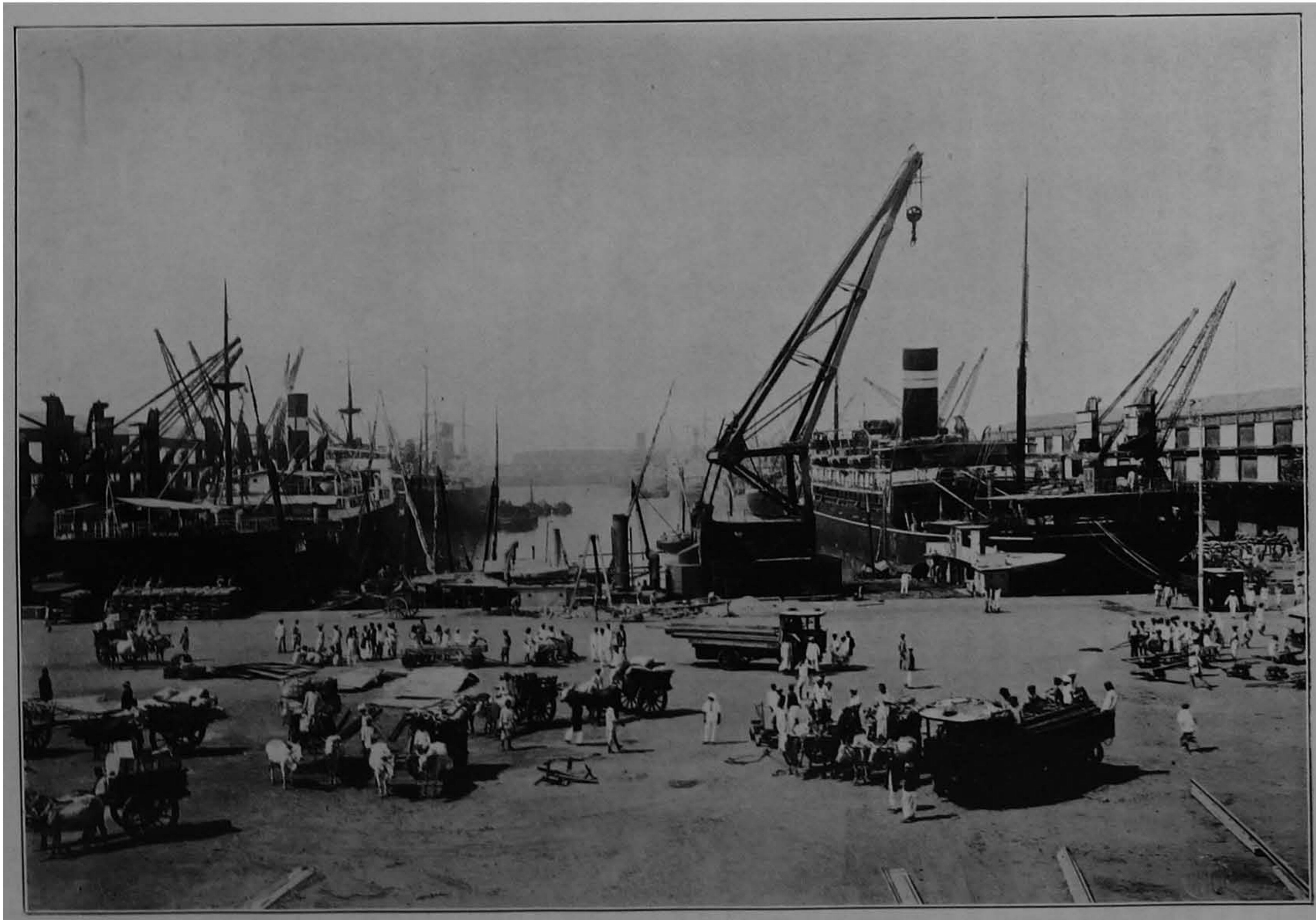
Shipping at the West and Jetty Wharves, Alexandria Dock, with the Port Trust 60-ton floating crane at work.
