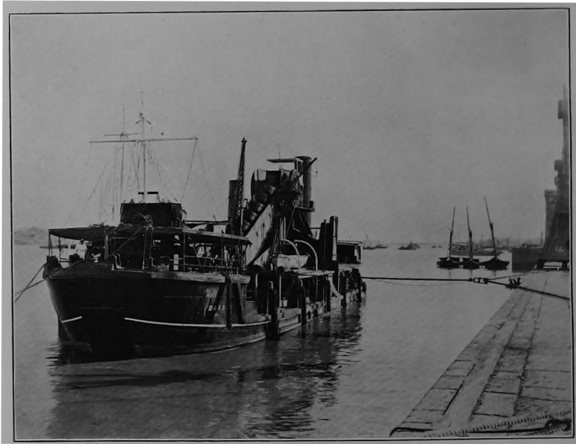
The Port Trust bucket ladder dredger "Barbus" at work off the Harbour Wall.
