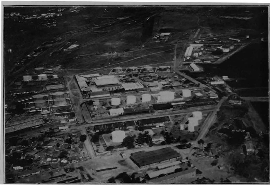
The kerosene oil installations.
