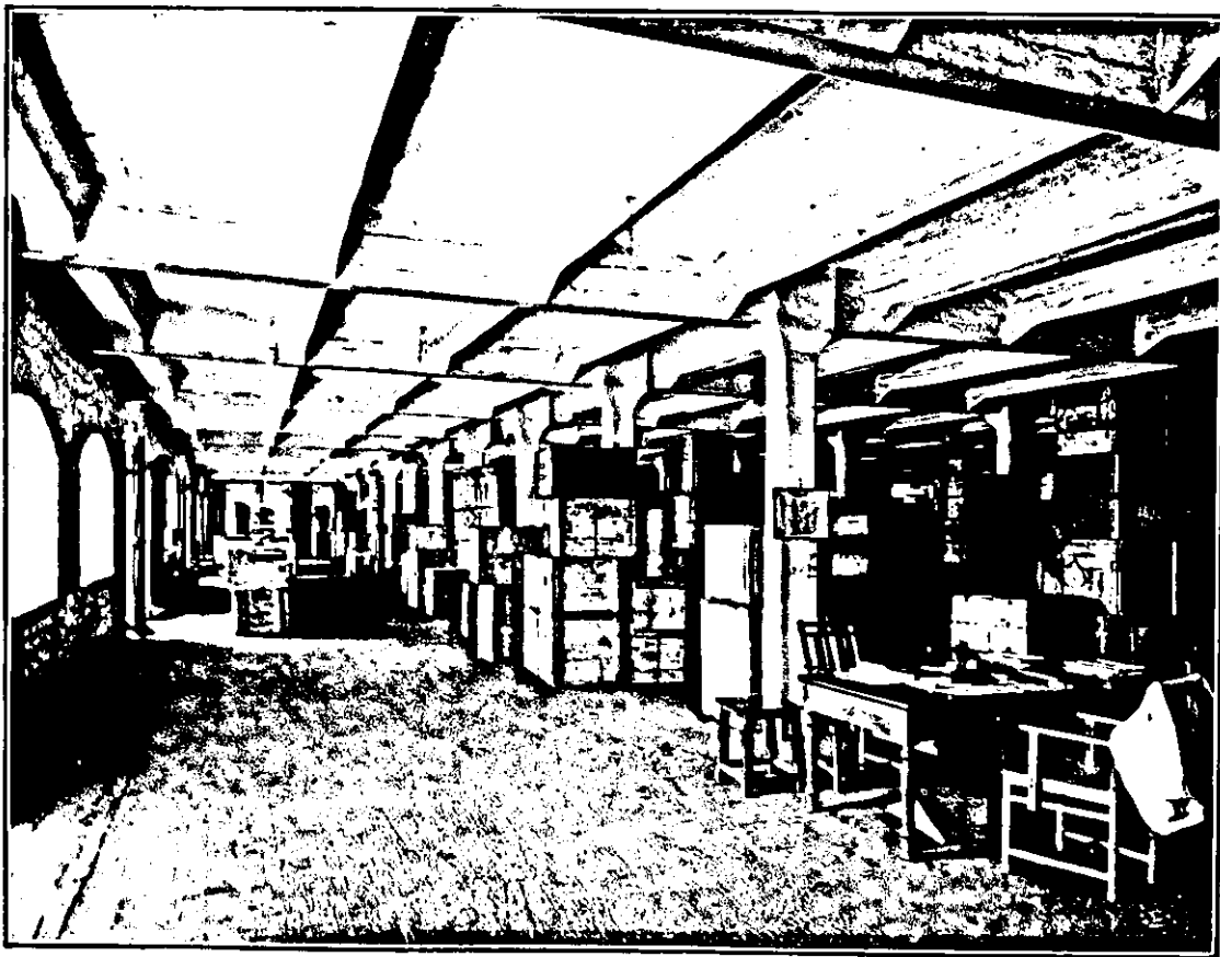
An upper floor interior, Alexandra Dock Warehouses.
