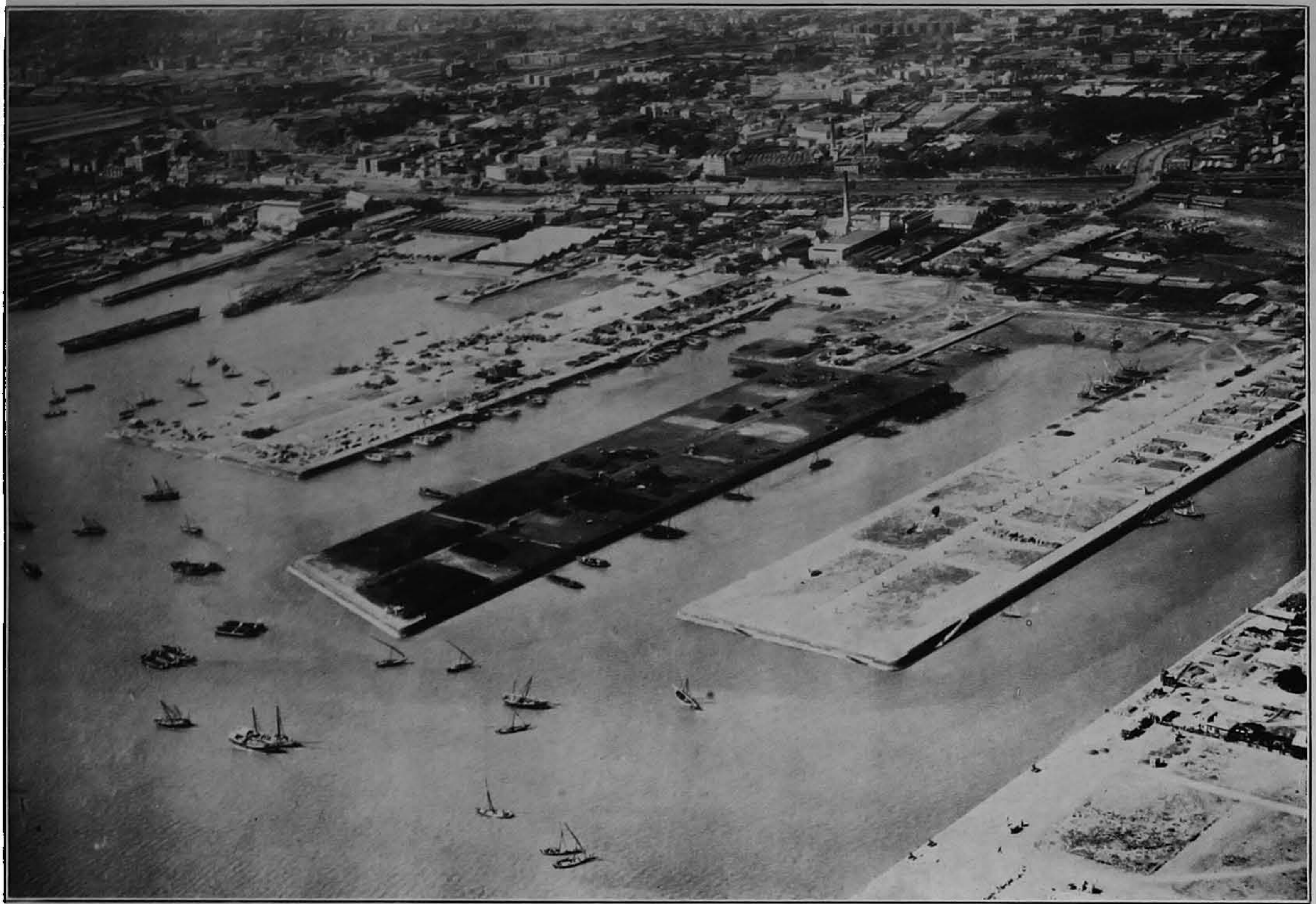
Some of the Port Trust bunders which accommodate the country boat traffic.
