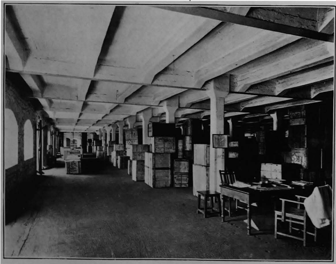
An upper floor interior, Alexandra Dock Warehouses.
