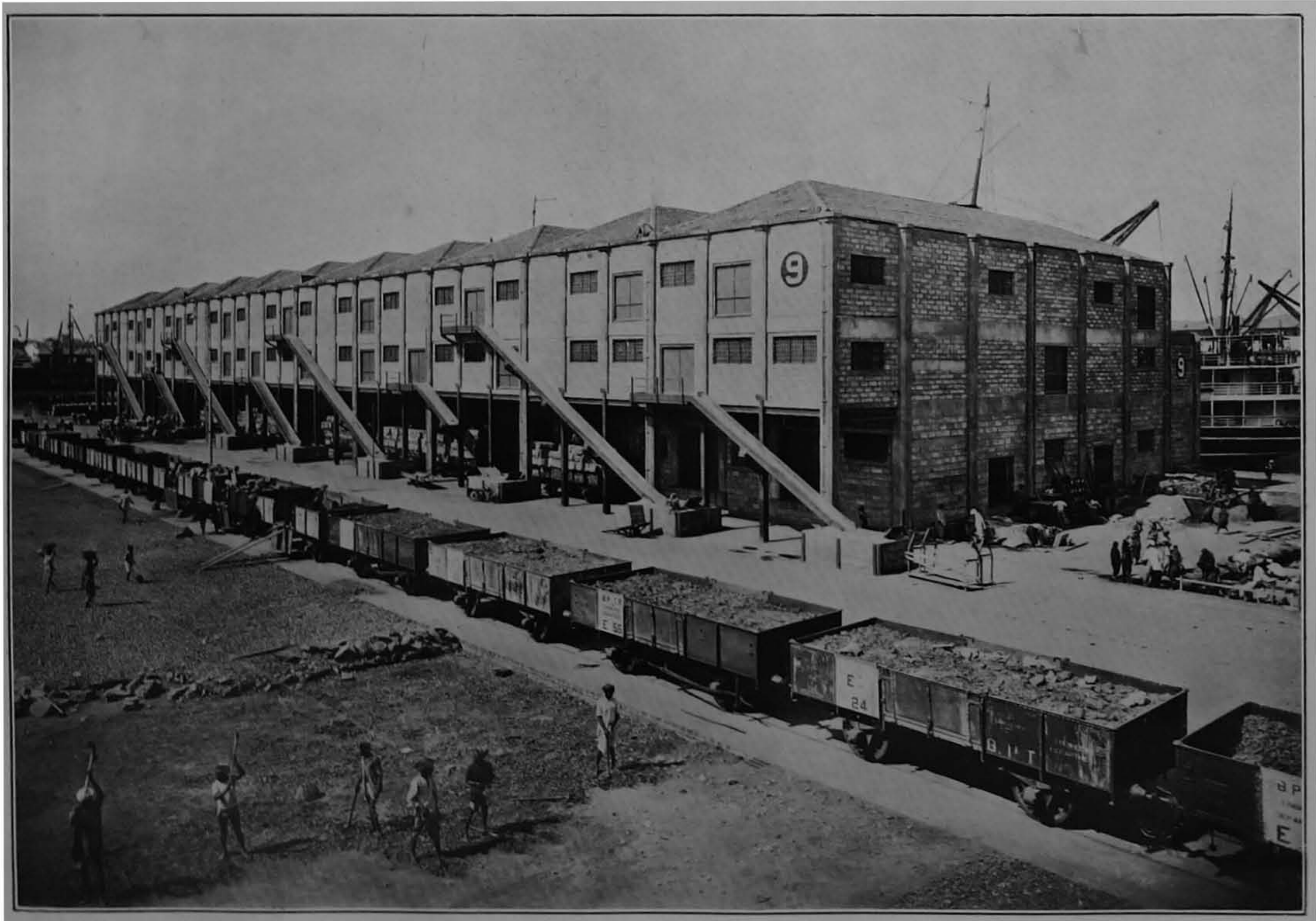
The latest type of dock transit shed, No. 9, Alexandra Dock ( exterior ).
