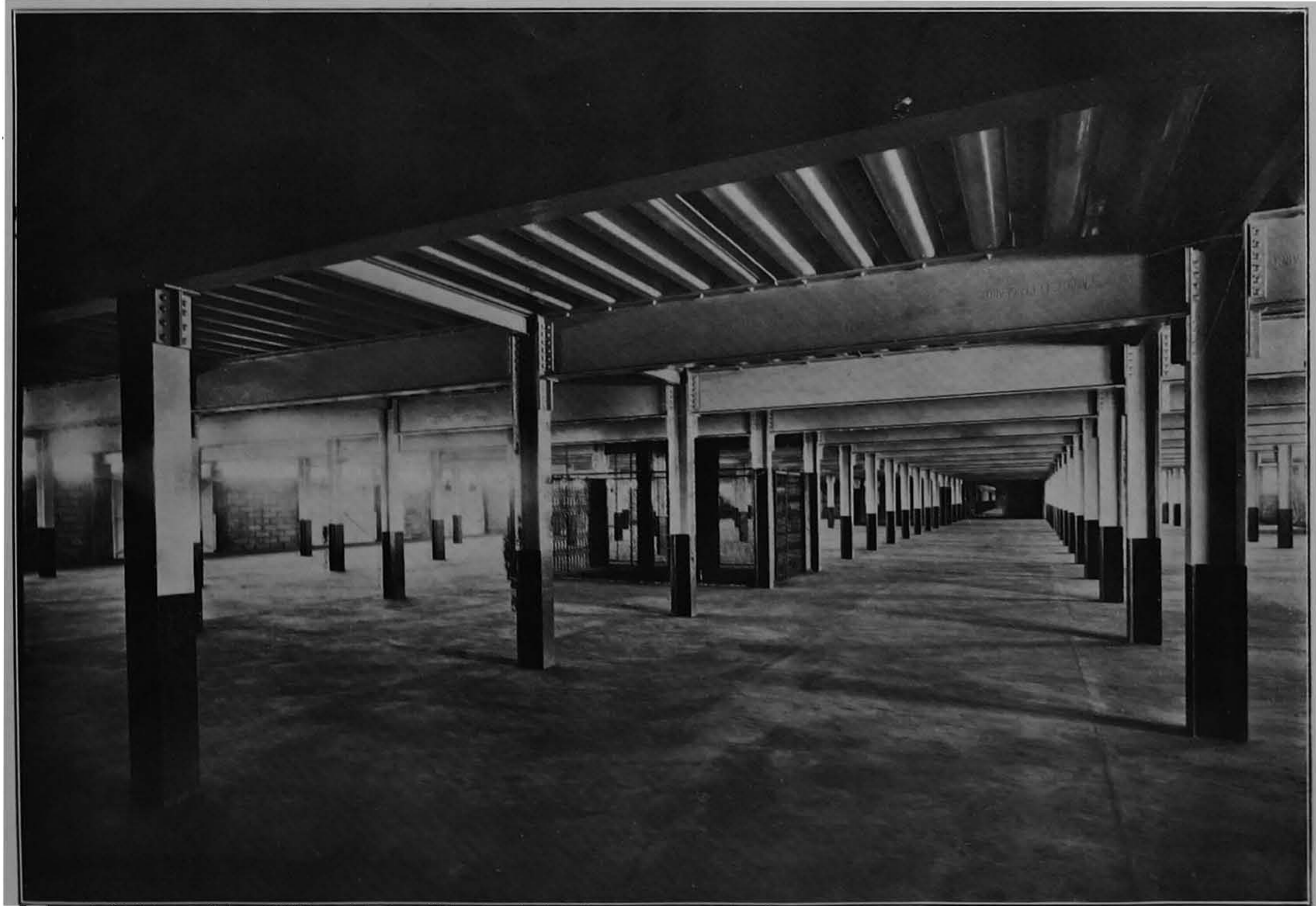
Transit shed No. 9, Alexandra Dock (interior, 1st floor).
