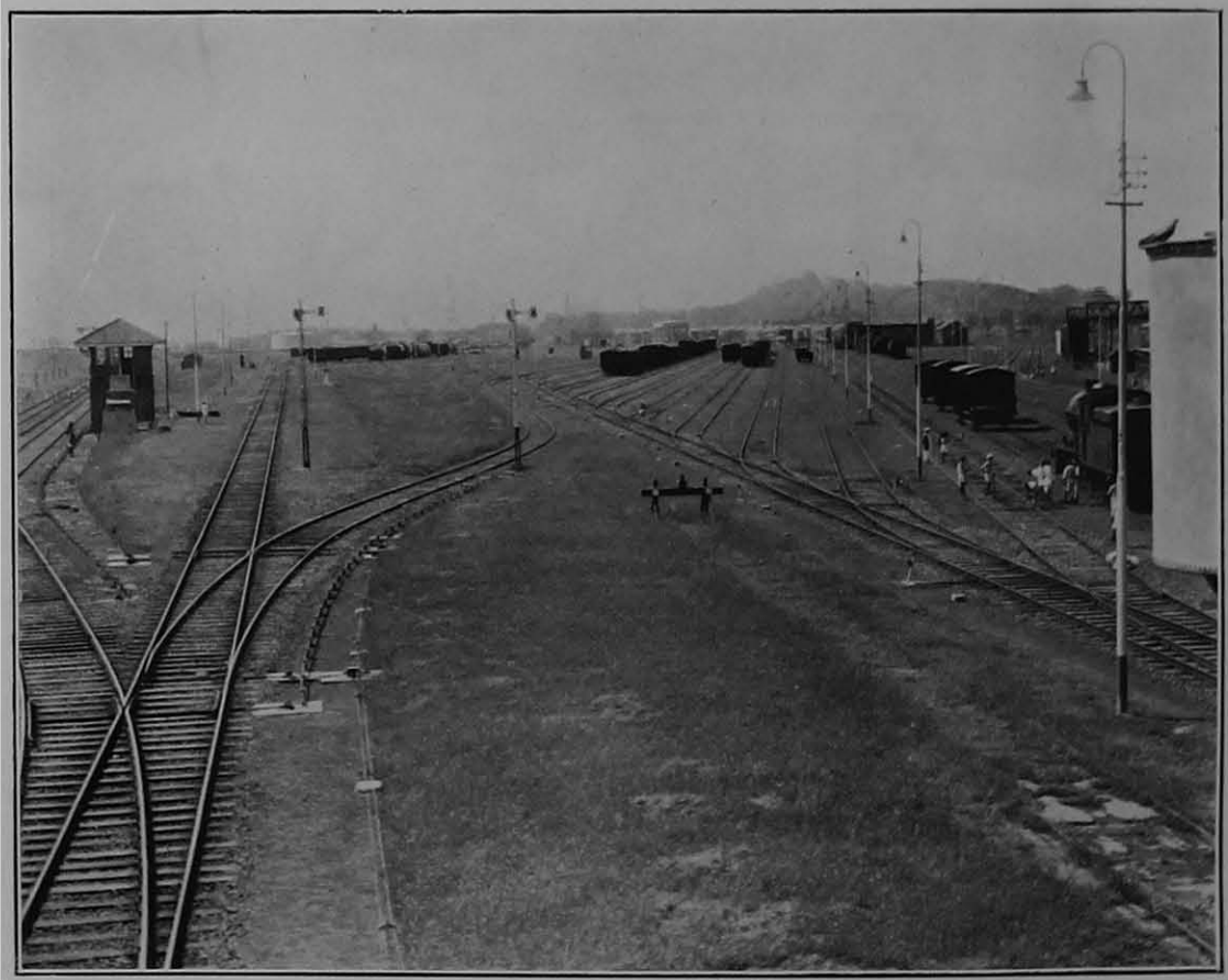
The Down Sorting Yard, Port Trust Railway, Wadala Junction.
