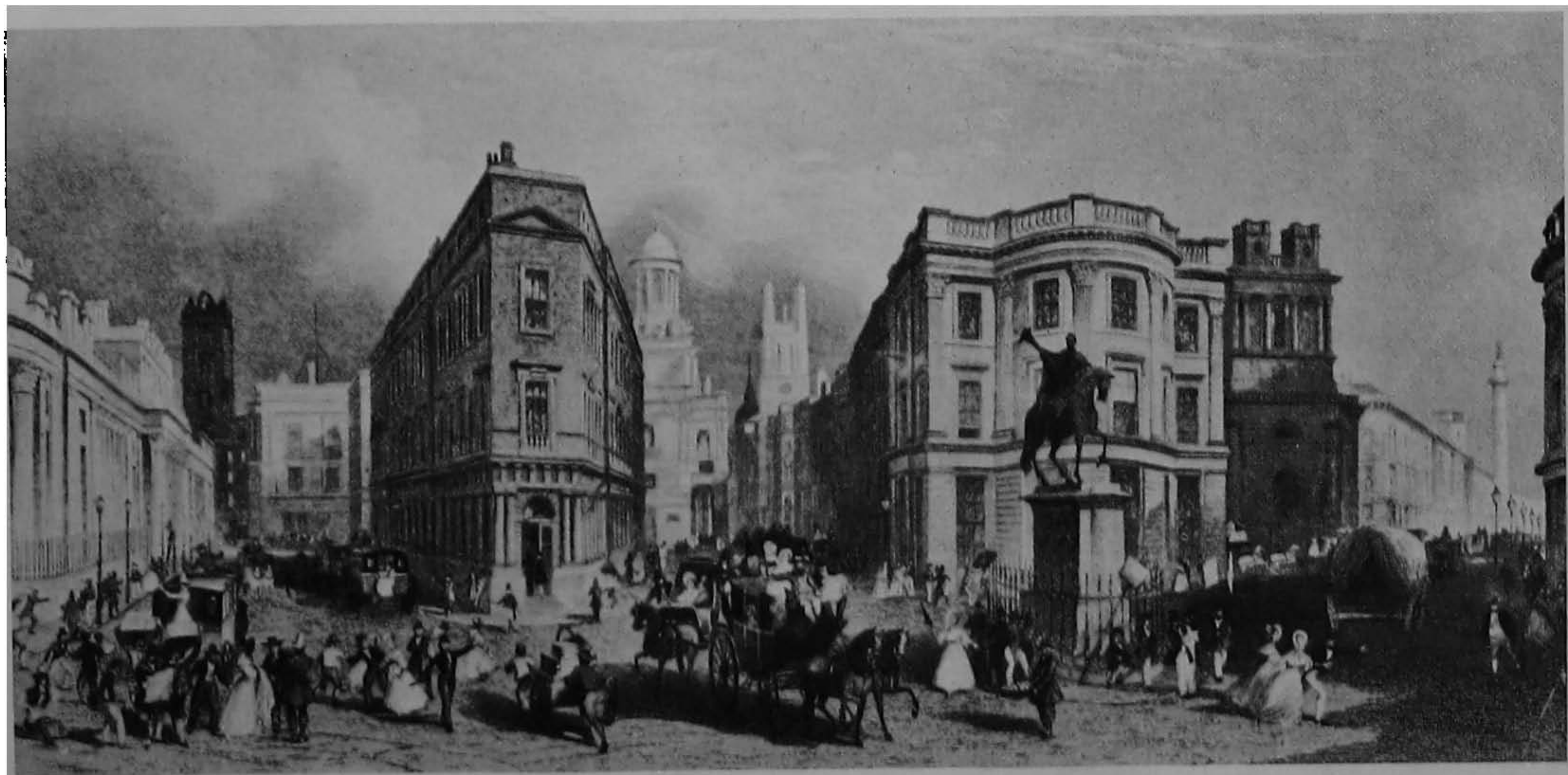
THE BANK AND MANSION HOUSE, KING WILLIAM STREET, 1850 .
