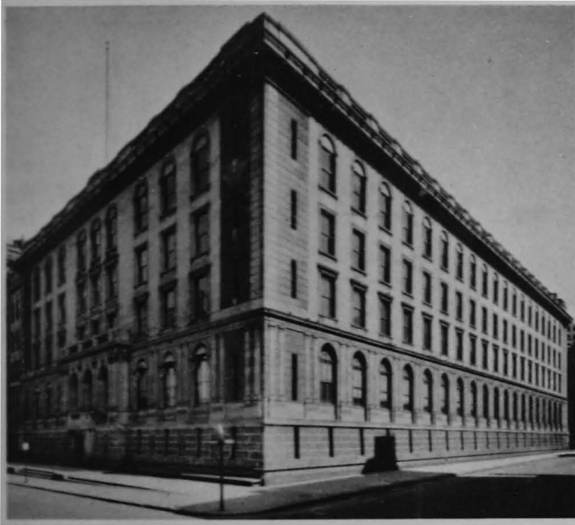
FEDERAL RESERVE BANK OF BOSTON 30 Pearl Street, Boston, Massachusetts
