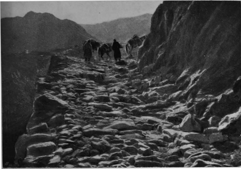
THE TRACK ALONG THE KOHRUT DAM.
